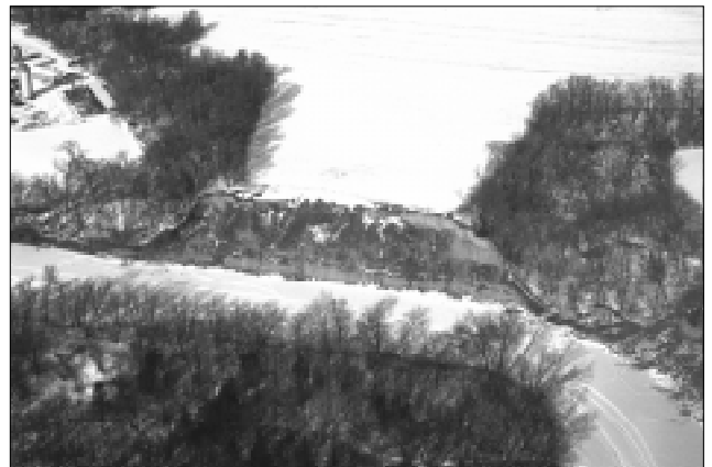
Stream bank erosion on the Blue Earth River.
