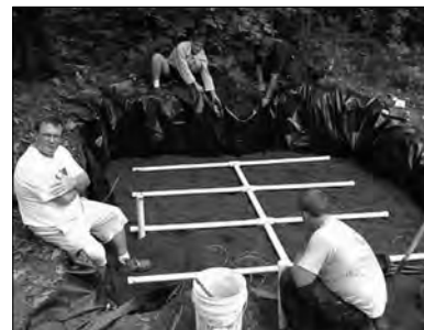
A recirculating sand filter distribution system is set in place.
