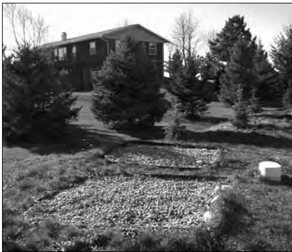
Recirculating sand filters at Lake Washington, MN.
