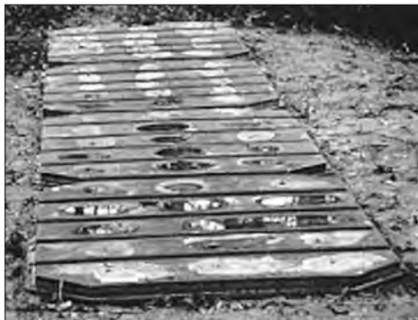
Installed prefabricated peat modules.
