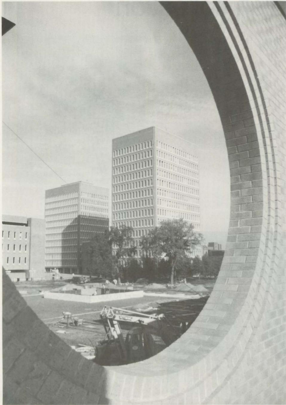
The circular brickwork on the second floor patio outside the reception room frames (left to right) Wilson Library, the Management/Economics Tower, and the Social Sciences Tower. The Music Library is under the plaza in front of Ferguson Hall.
