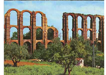
Top: the Pont du Gard, built ca 19 BCE, using massive cut stones and no mortar. Maximum height is 47 m. Bottom: Los Milagros aqueduct (late 1st Century), near Merida Spain. Concrete with stone facing; height 25 meters.
