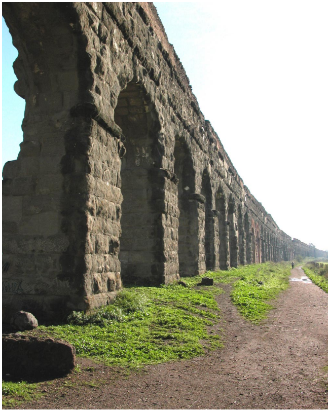
The "Acquedotto Claudio" was initiated by Caligola in 38 AD and completed by Claudius in 52 AD (it was likely active already in 47 AD). The aqueduct had a total length of ca. 69 km, the last 9.5 km of which were built over arches (the initial part was underground). The aqueduct is relatively well preserved. Here the height ~17 m and the distance between pillars is 5.5 m. The pillars are made of local tuff blocks (volcanic products from the Alban Hills), slightly cemented. (photo by Leonardo Sagnotti).
