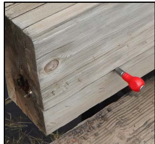
Figure 4.2. An awl is used to assess the depth and presence of decay in a horizontal split.
