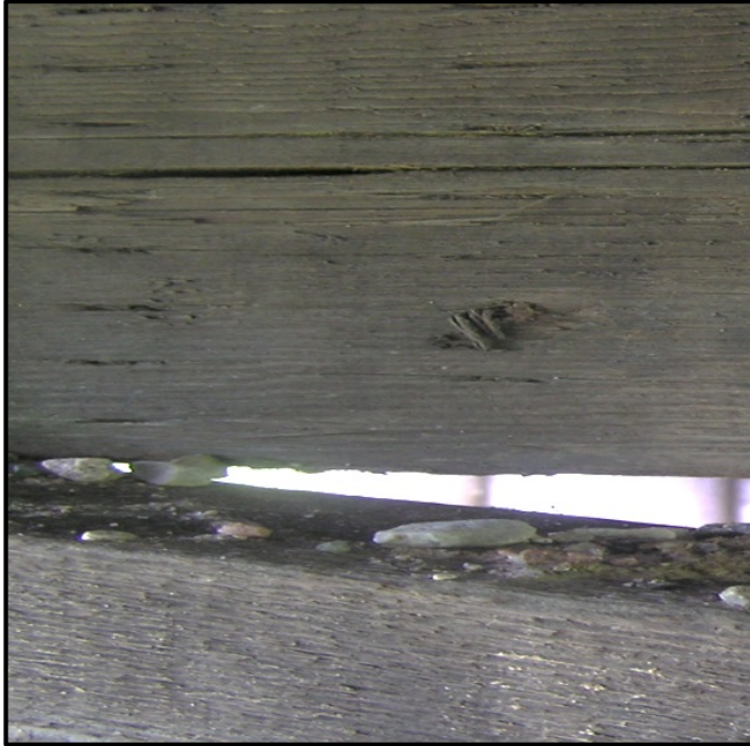
Figure 3.8. A timber abutment cap that has been initially deteriorated by decay. Carpenter ants are nesting in the cap, with frass being deposited onto the cross bracing member.
