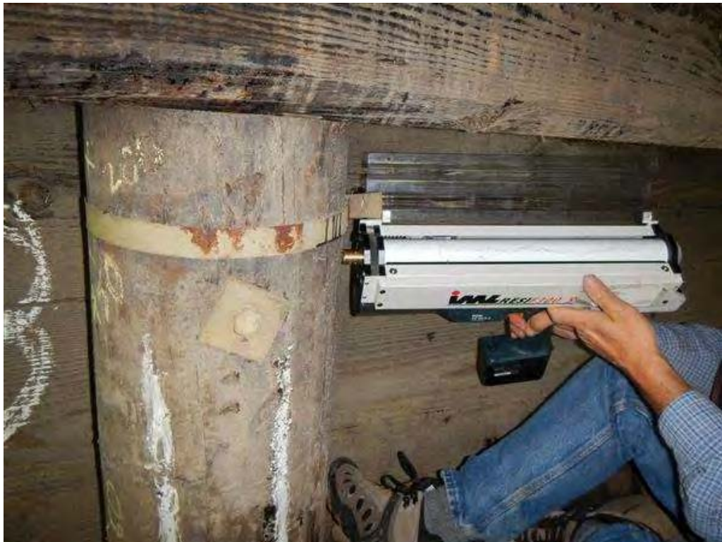
Photo 14 - E abut - Pile 11 - Sound condition
