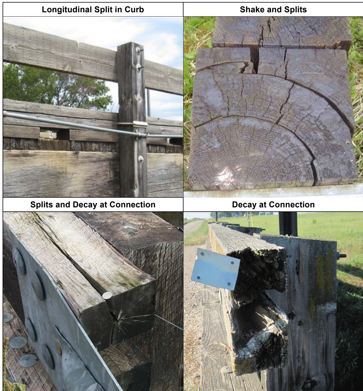
Figure 7.4. Examples of deterioration of timber railing components.
