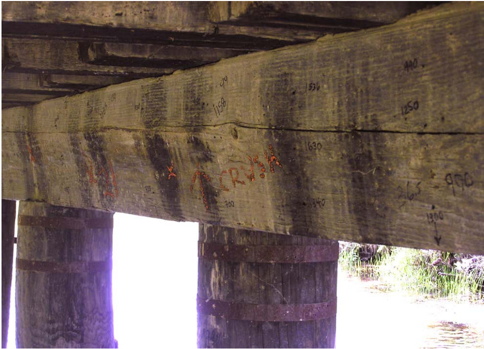
Figure 3.13. A long horizontal split provides an opportunity for moisture passing through the timber deck to enter the abutment cap, leading to substantial decay.
