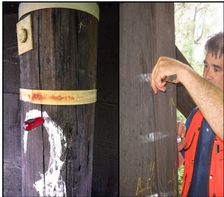
Figure 4.3. Probes are used to assess the depth of cracks, checks and through splits in timber bridge elements.
