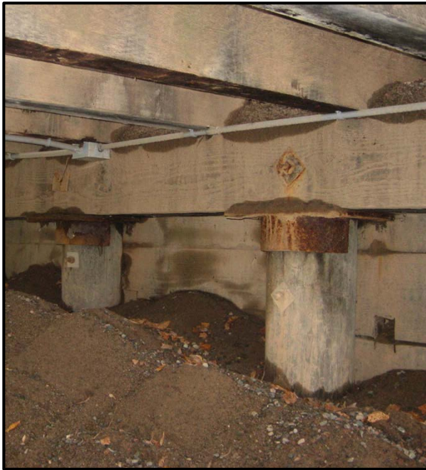
Figure 3.21. Sand and gravel are shown on top of the timber abutment cap as deposited through vehicle traffic or road maintenance through a timber deck.
