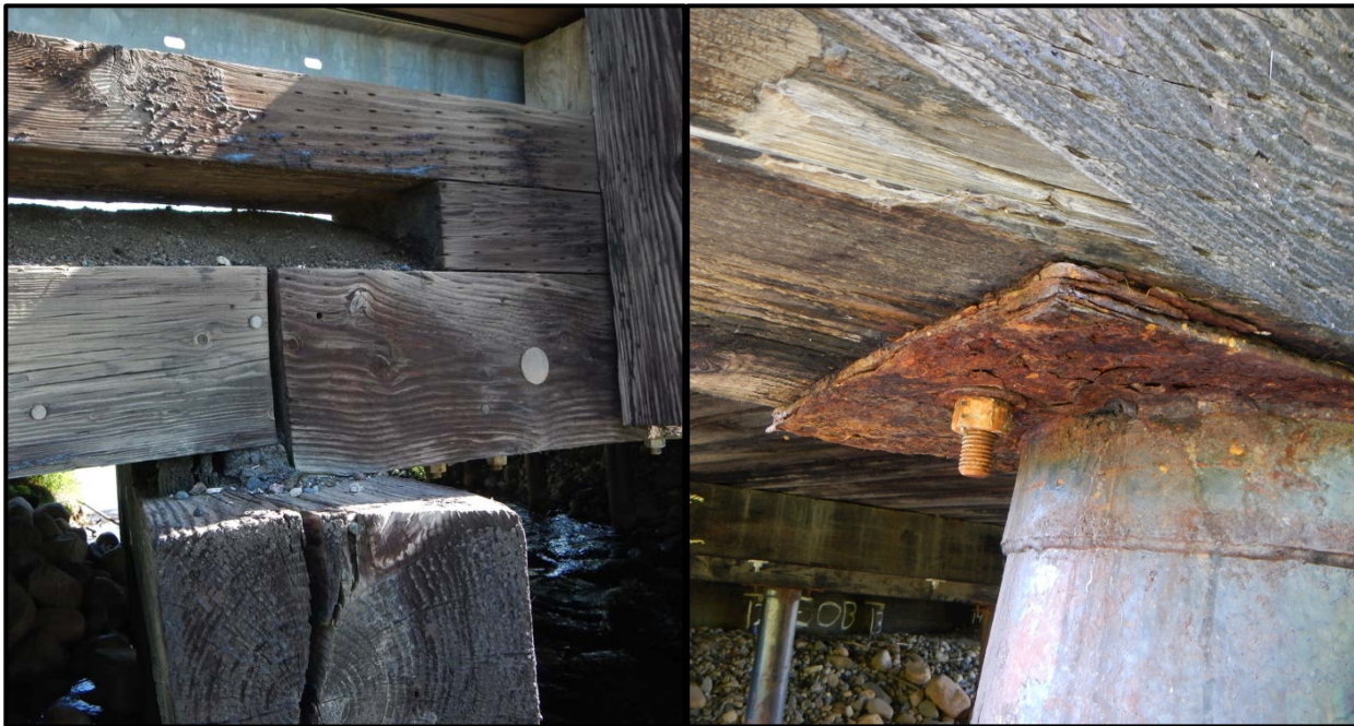
Figure 3.14. Visual assessment of a pier cap split. The split allows moisture from the deck to enter the member beyond the protective layer of preservative treated wood, resulting in increased likelihood of future decay and allows for deterioration of hardware such as the CIP bearing plate that supports this element.
