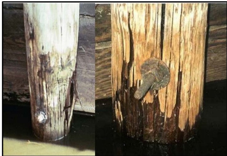
Figure 3.18. Shell damage to timber piling at or near the water line, often caused by freeze thaw cycles, ice damage or flotsam floating down the river.
