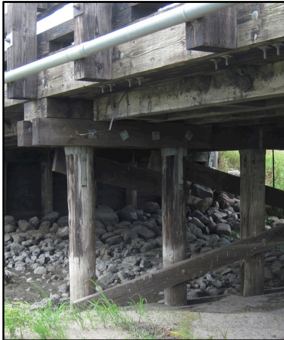
Figure 1.7. Timber piling and cap materials forming an intermediate support pier.
