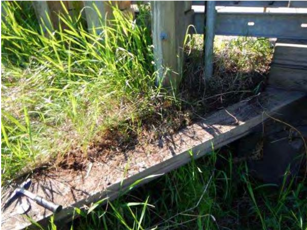
Photo 16 - Wing wall - NE
