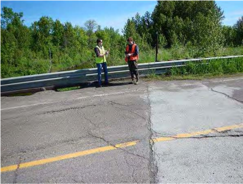
Photo 3 - Bituminous east end before abutment
