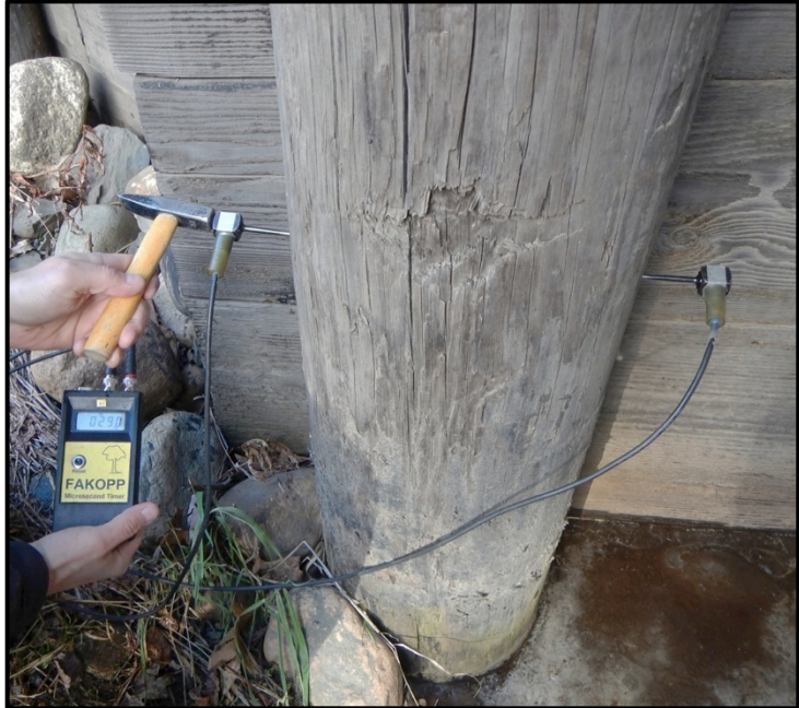
Figure 5.2. A stress wave timer is used to determine the level of decay in a timber piling.
