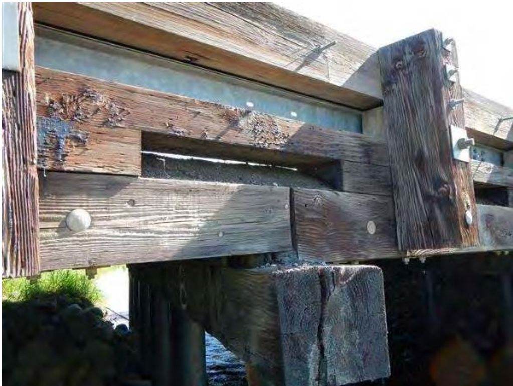
Photo 10 - Pier 2 North end - Through split extending 14" into cap.
