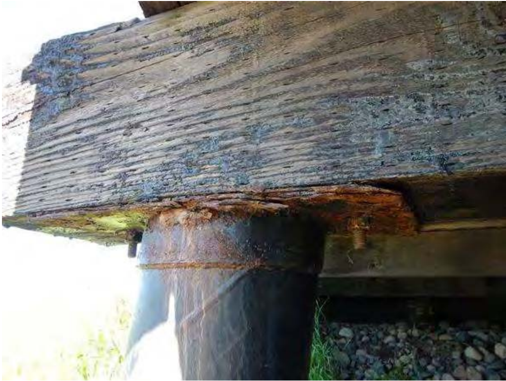
Photo 13 - Pier 1 -CIP cap plate rusting with section loss.
