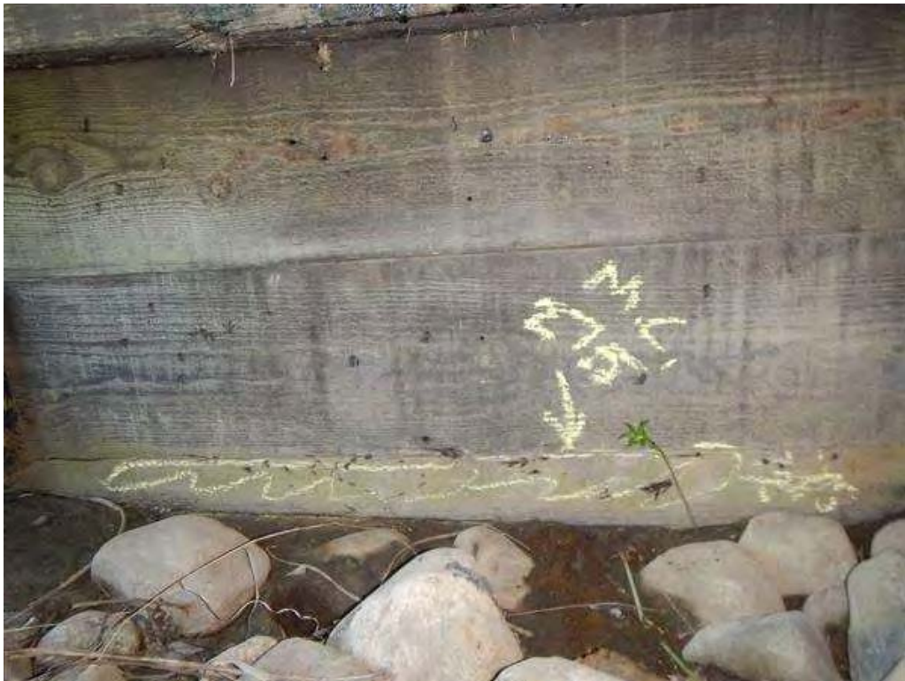
Photo 12 - High moisture abutment wall between piles 8 and 9. Moisture content over >25% but no decay present.
