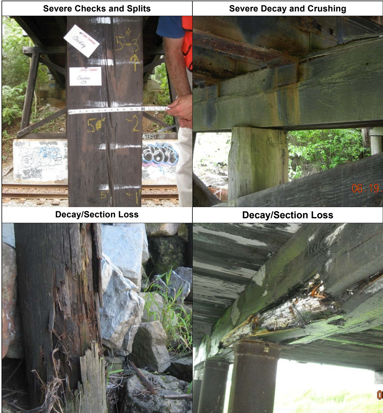
Figure 7.7. Examples of deterioration of timber substructure elements.
