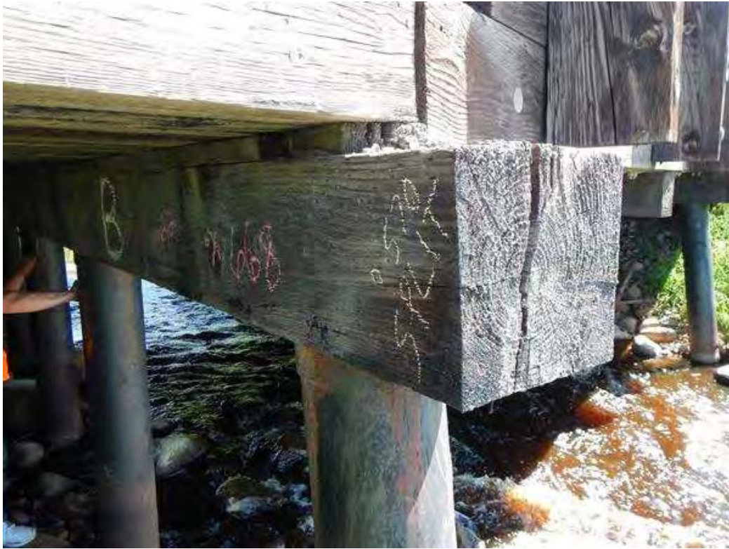
Photo 7 - Pier 1 - South End - Through split extending 36"
