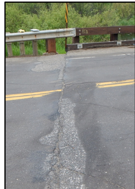
Figure 3.15. Transverse cracking that occurs over the beginning of bridge abutment.
