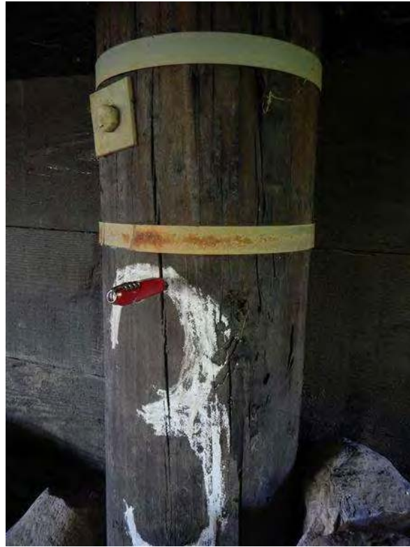
Photo 11 - W. Abut. Pile 3
