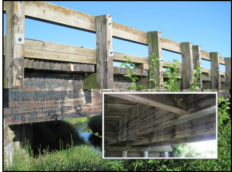
Figure 1.2 Glulam beam timber bridge construction.
