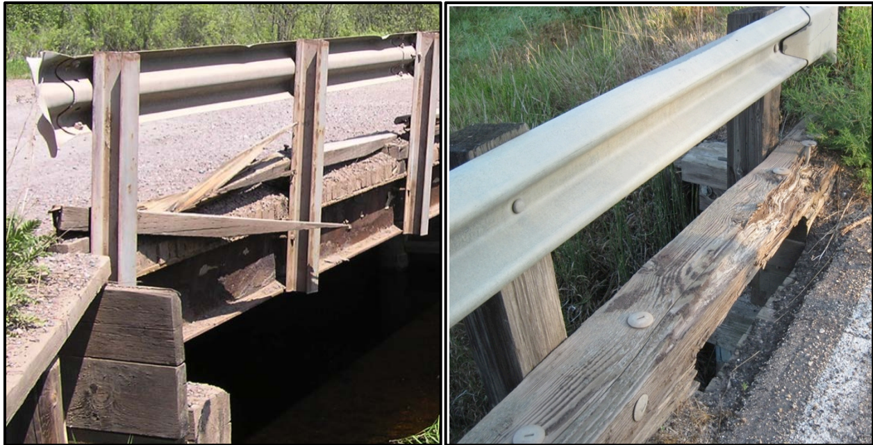
Figure 3.19. The timber curbs shown have significant damage from a snowplow or other vehicle exposing untreated wood to high levels of moisture.
