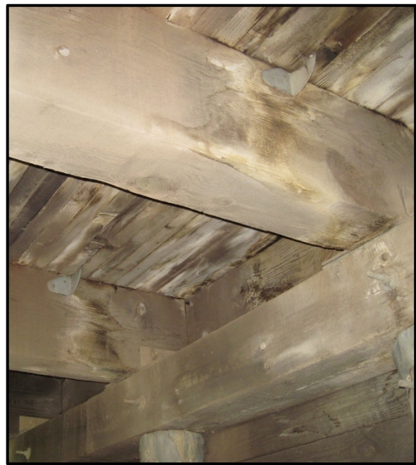
Figure 3.7. Water staining and discoloration caused by water that infiltrated through the bituminous wear layer and nail-laminated deck.
