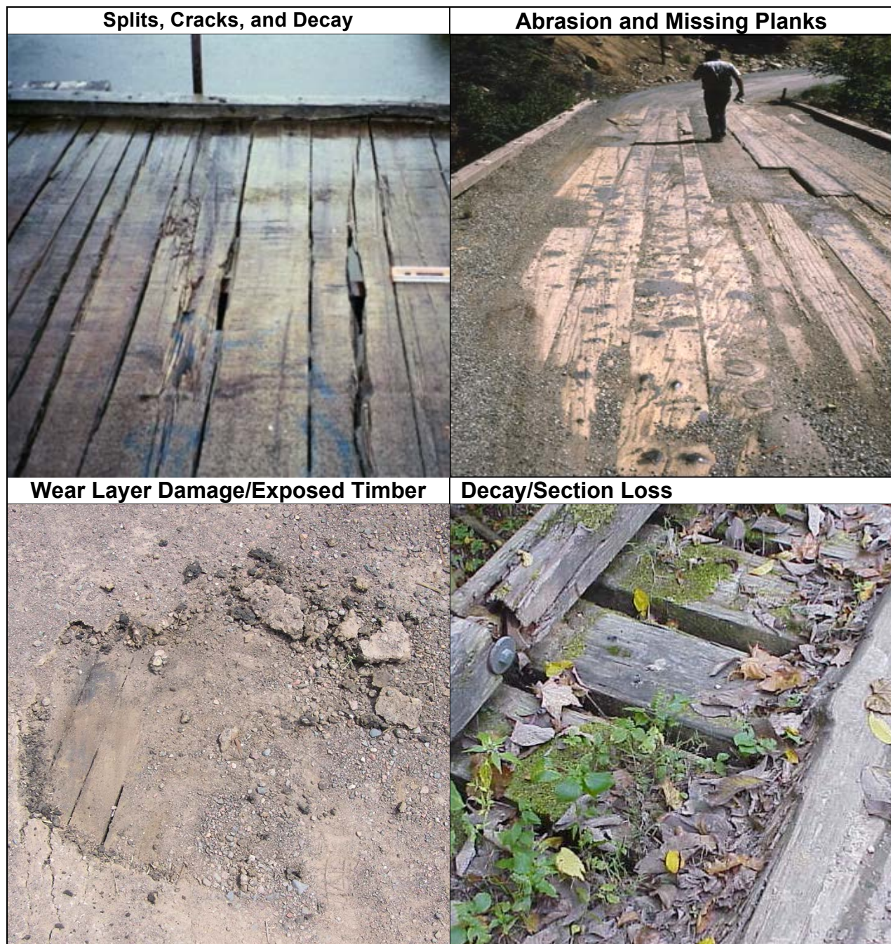
Figure 7.3. Deterioration of timber decks and slabs.
