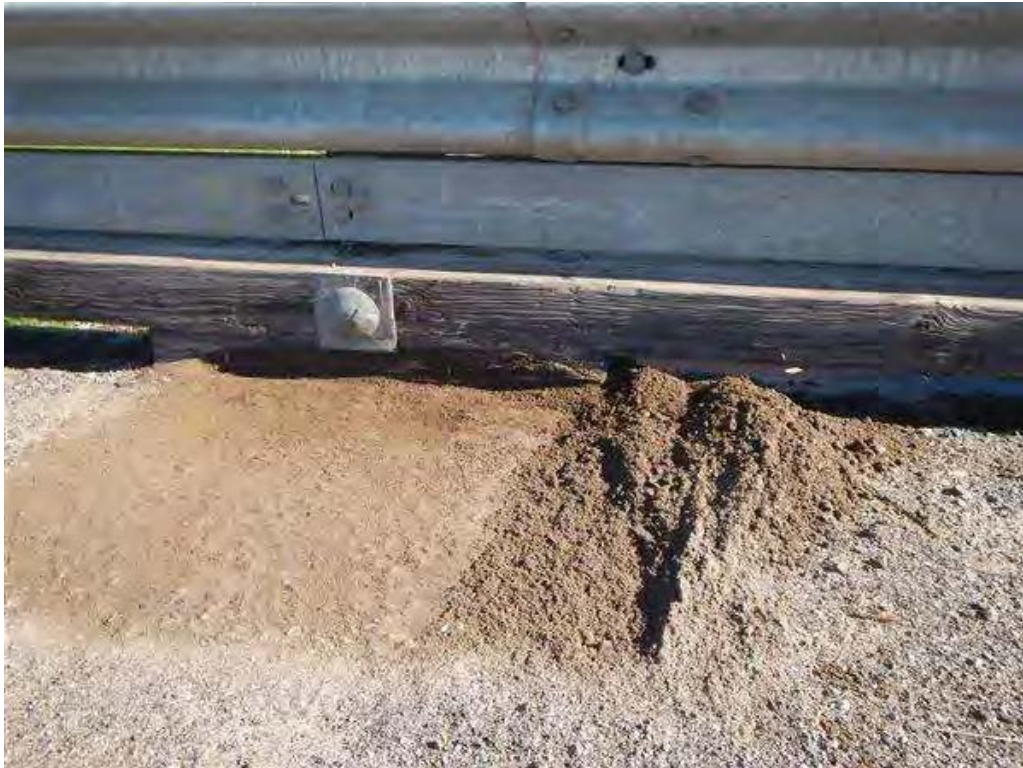
Photo 4 - N. deck-scupper 3" sand on deck
