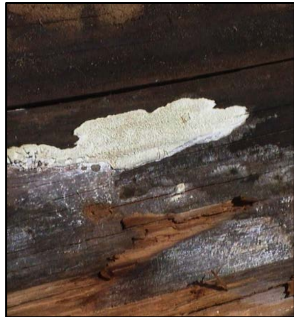
Figure 3.2. Douglas fir bridge member showing visual evidence of a fruiting body on the surface in addition to visual evidence of decayed timber.
