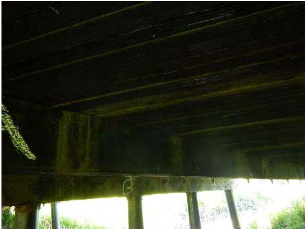
Photo 8 - Span 1 - Moisture pen. through deck.
