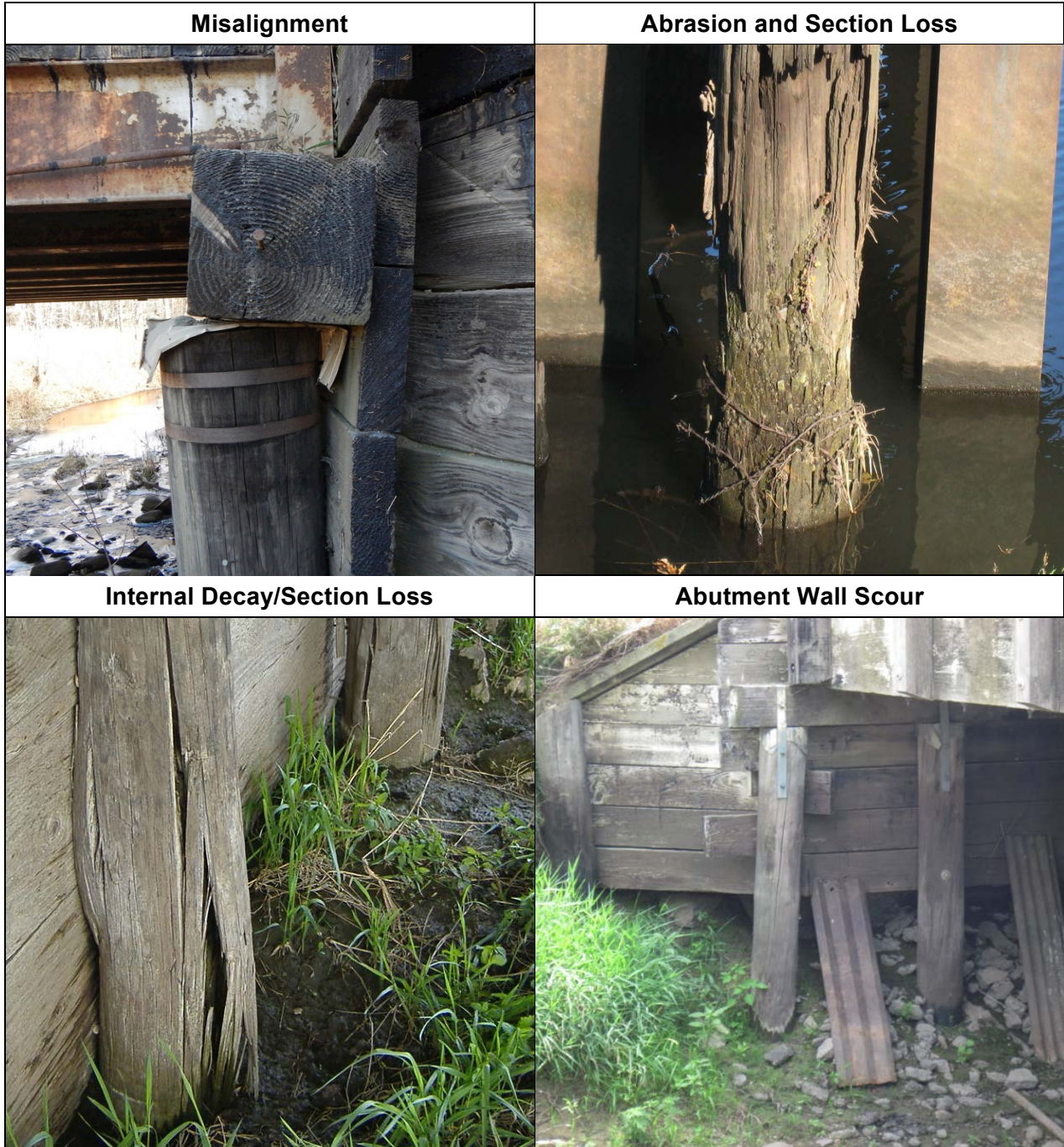
Figure 7.6. Examples of deterioration of timber substructure elements.
