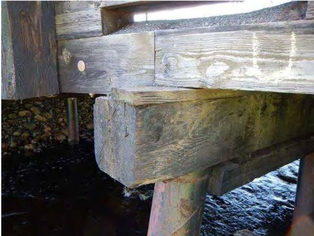
Photo 6 - Pier 1 - North End - Through split extending 80% of full length of cap. SWT over 500 but R drill showed only crack with no decay
