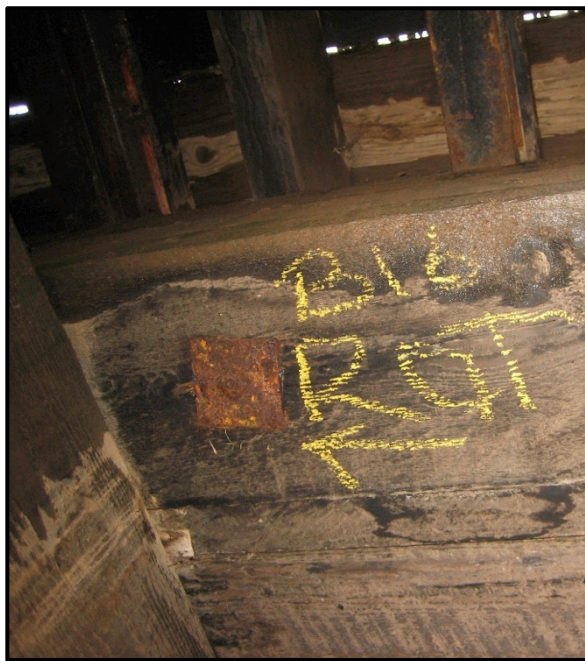
Figure 3.6. The timber members were stained and discolored due to high levels of water. The hardware shows significant corrosion.
