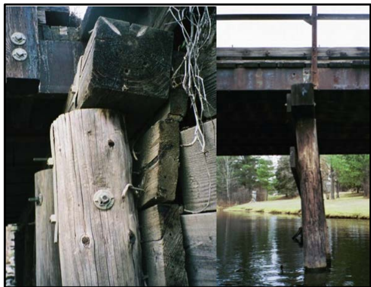
Figure 3.20. Rotation of timber pilings and pile caps in an abutment (left) and timber pier (right).
