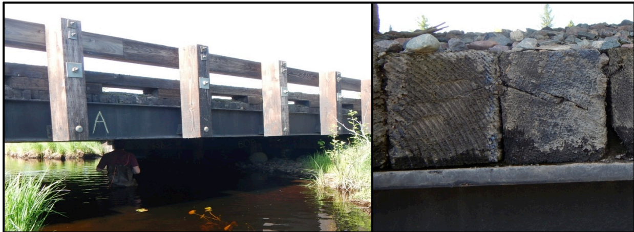
Figure 1.3. Steel beam bridge with a nail laminated timber deck.
