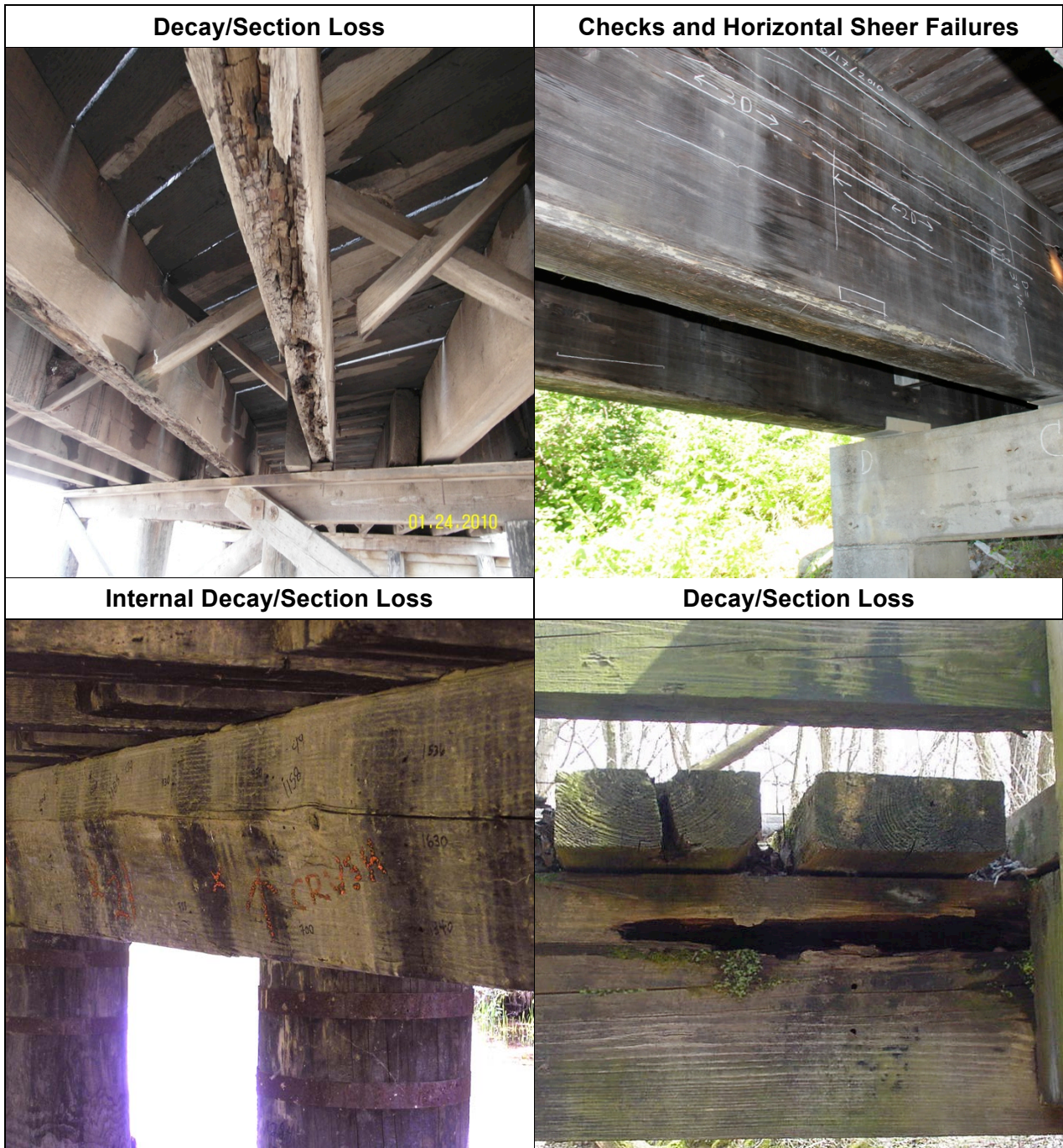
Figure 7.5. Examples of deterioration of timber superstructure elements.
