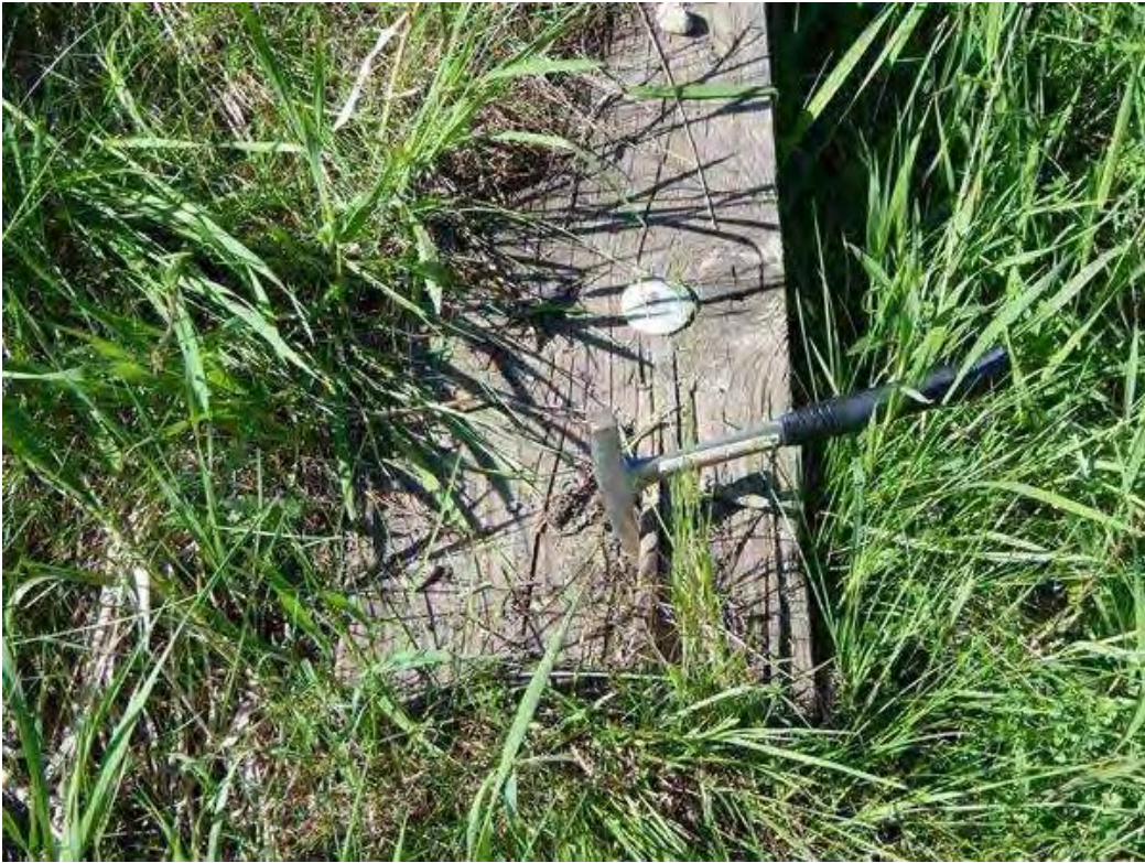
Photo 15 - Wing wall - NE
