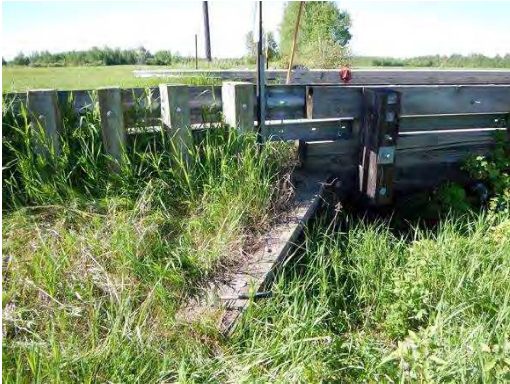
Photo 17 - Wing wall with significant vegetation
