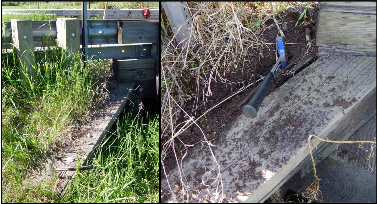
Figure 3.11. A wing wall timber abutment has substantial plant growth on the cap surface. Once removed, visual and probing inspection showed that 75% of the cap cross-section had been severely decayed. This will eventually result in damage to the wing wall pile elements.
