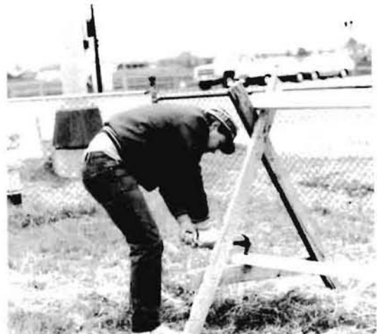
The start of the Green Hall addition.
