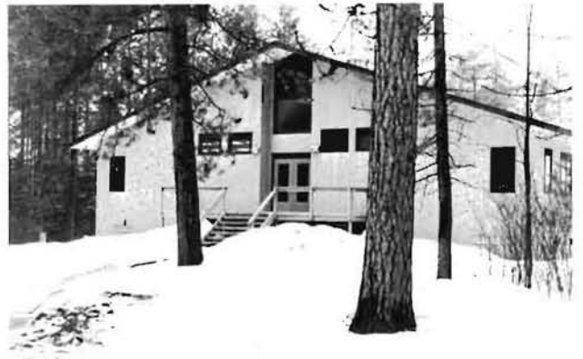
New Classroom Building, Cloquet Forest Research Center
