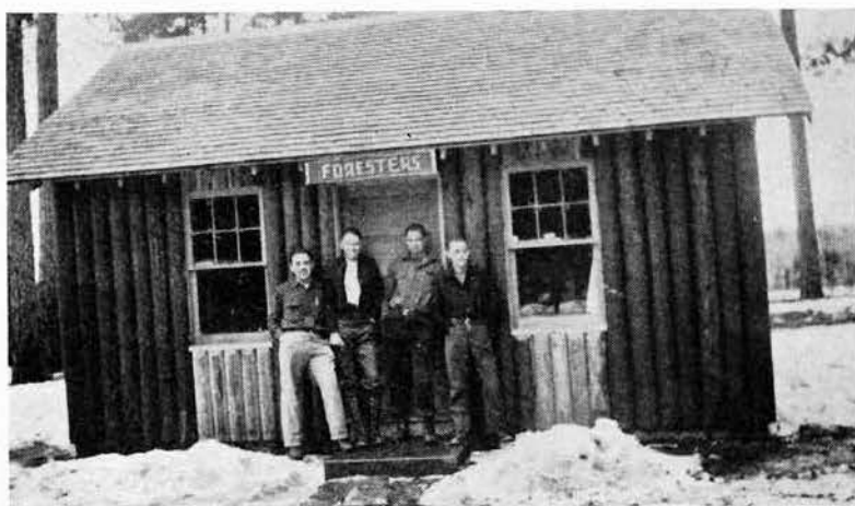
"The foresters cabin was in an advantageous position, being closest to the cook shack."
