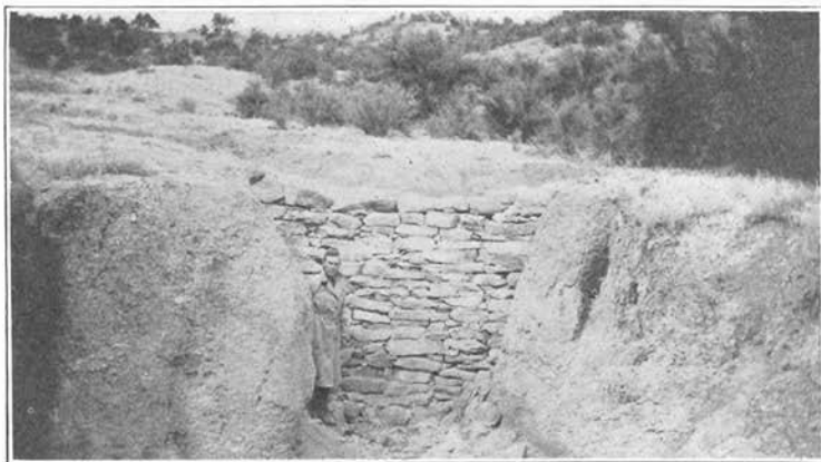
A typical erosion check dam.
