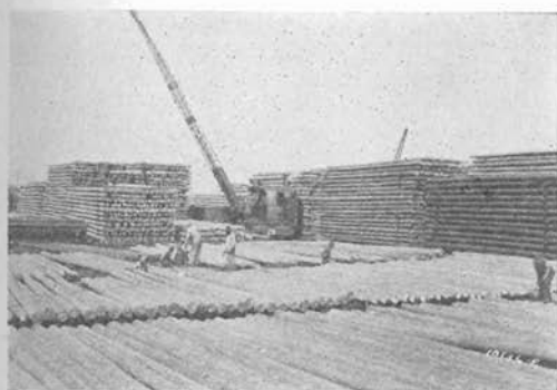
A modern pole yard.
