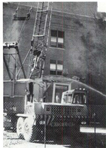
Demolition of the former Zoology and Botany buildings was completed in November, making room for the new building.
