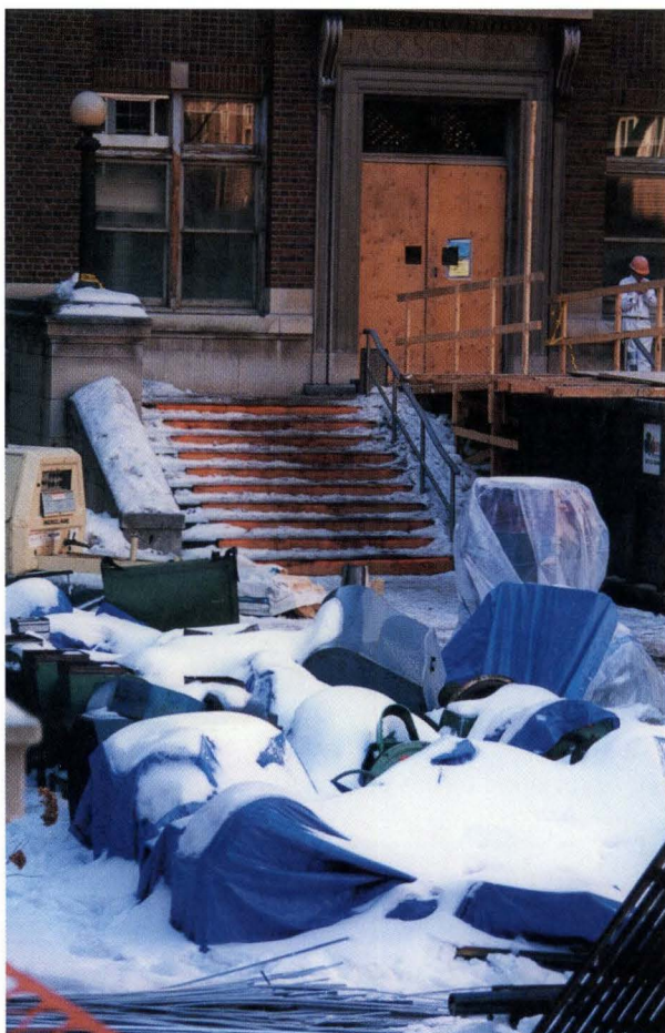
Refurbished Jackson Hall will house the new physiology lab.
