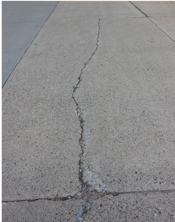
Figure 2.1: Schematic of a longitudinal crack (top) and photo of longitudinal cracking on a low volume road in Minnesota (bottom)(photo courtesy of Andrew Lederle)
