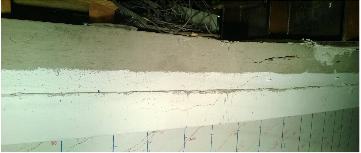
Figure C-38: Deck crushing observed during 36M_8W test.
