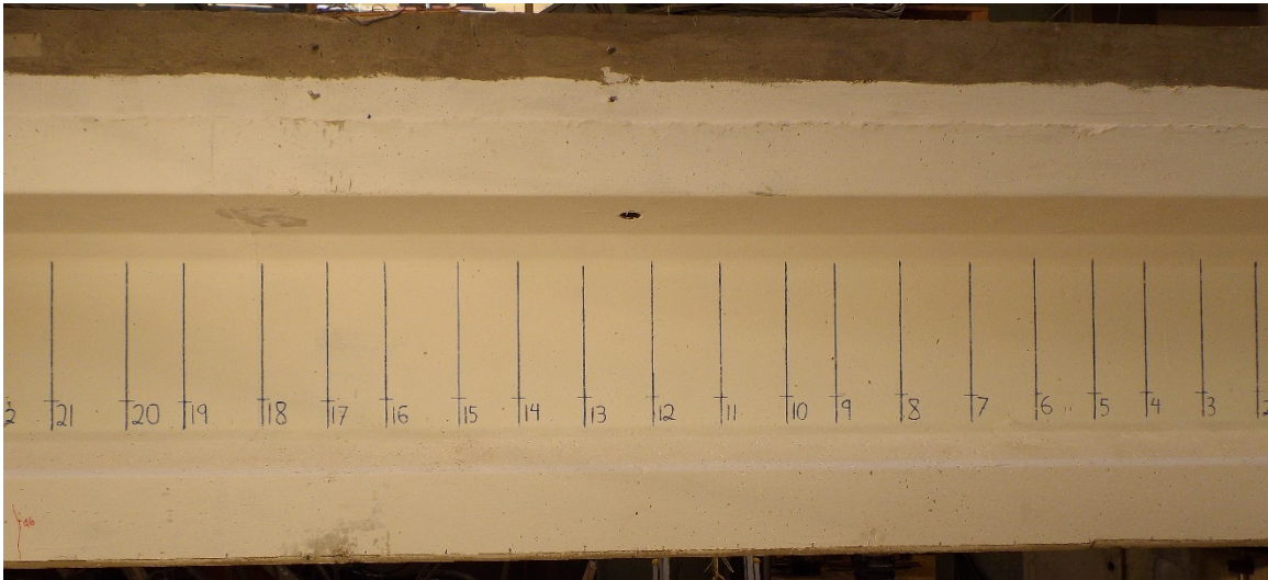
Figure C-18: Observed cracking in web-shear controlled region of 36M_18F test with 136.5 kips applied.
