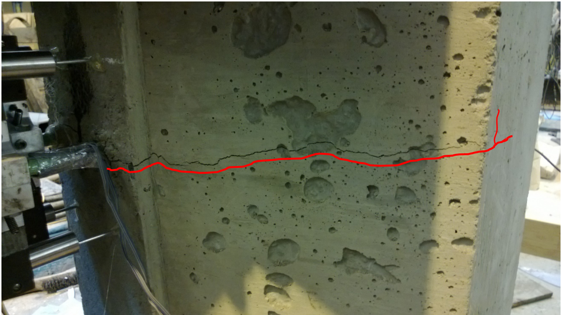
Figure 2-18: 8.0M_WC_20A splitting cracks at failure on the angled face of the flange representative of typical concrete splitting failure with minimum applied compressive force.
