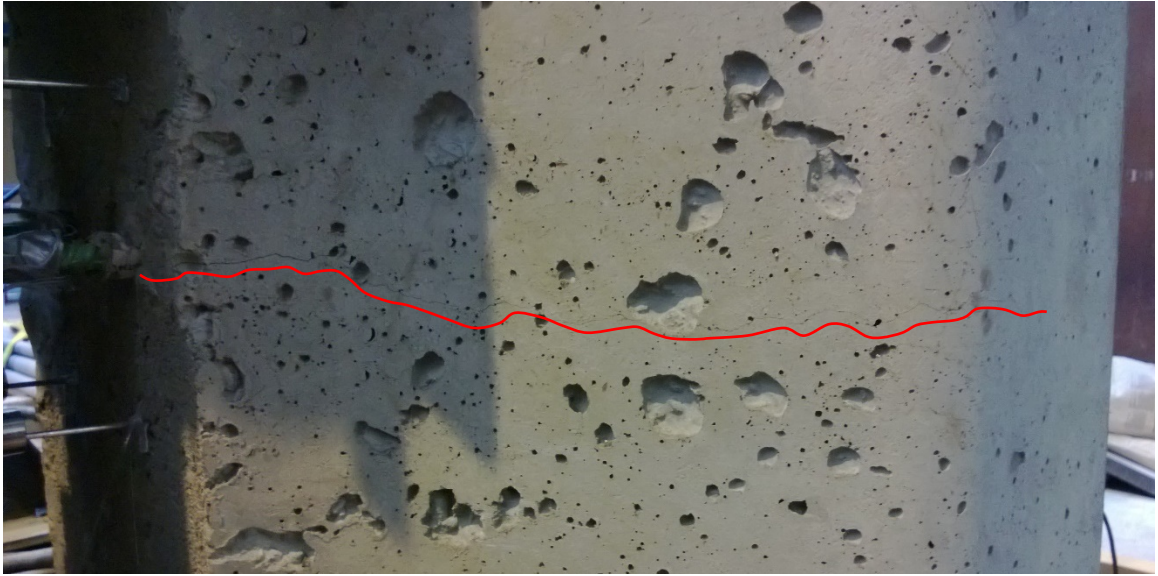
Figure 2-20: Splitting cracks following test of 8.0MN_WC_30A test which formed prior to bar fracture.
