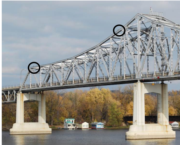
Figure 16: Bridge 5900 - Solar Panel Locations
