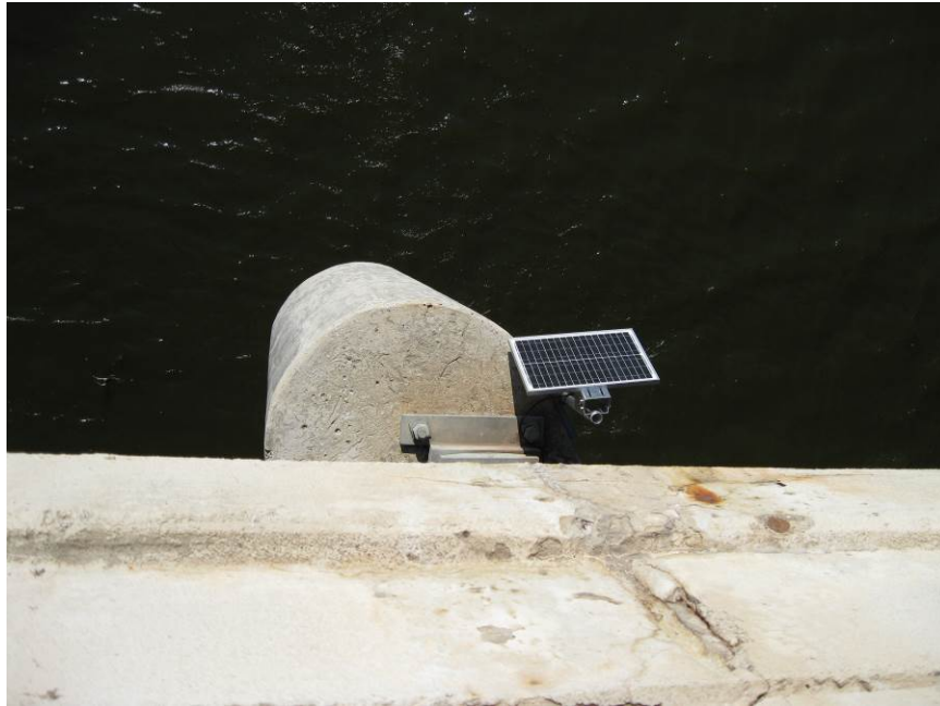
Figure 20: Bridge 07011 - Pier 4 Solar Panel
