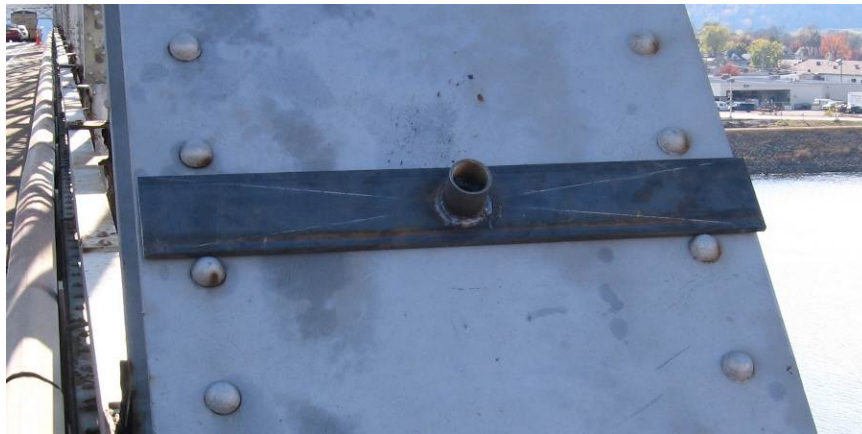
Figure 17: Bridge 5900 - Solar Panel Bracket
