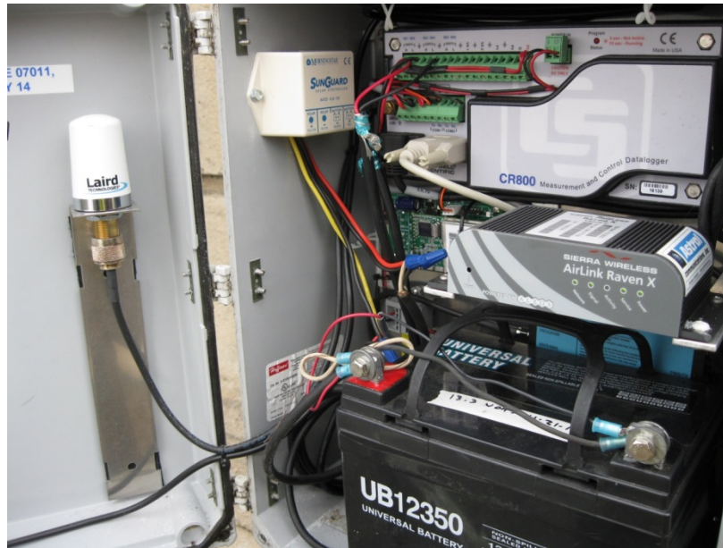
Figure 56: Relocated Solar Regulator
