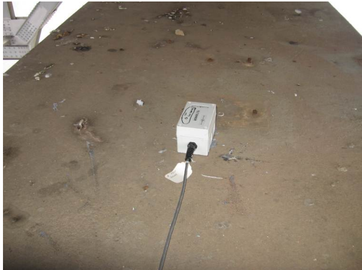
Figure 11: Bridge 5900 - Pier 20 Tilt Sensor
