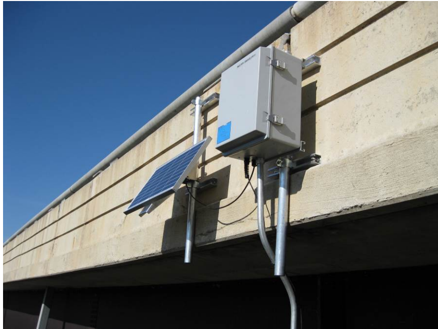
Figure 21: Bridge 07011 – Pier 5 Datalogger and Solar Panel
