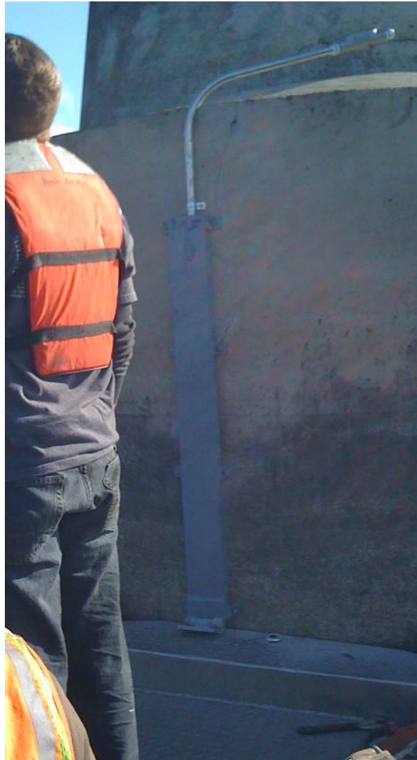
Figure 6: Bridge 5900 - Upper Sonar Mount
