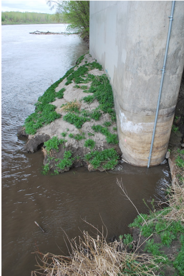
Figure 26: Pier 5 during 5/13/2014 Testing Event
