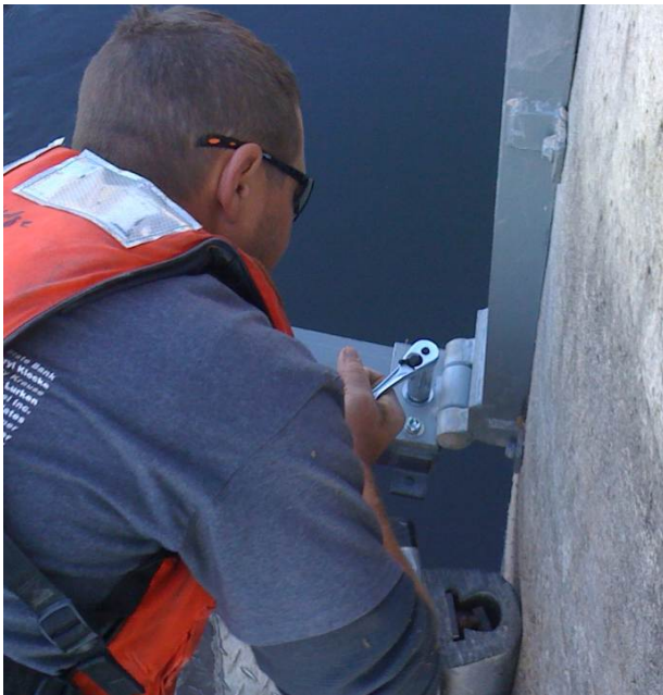
Figure 8: Bridge 5900 - Attaching Lower Mount
