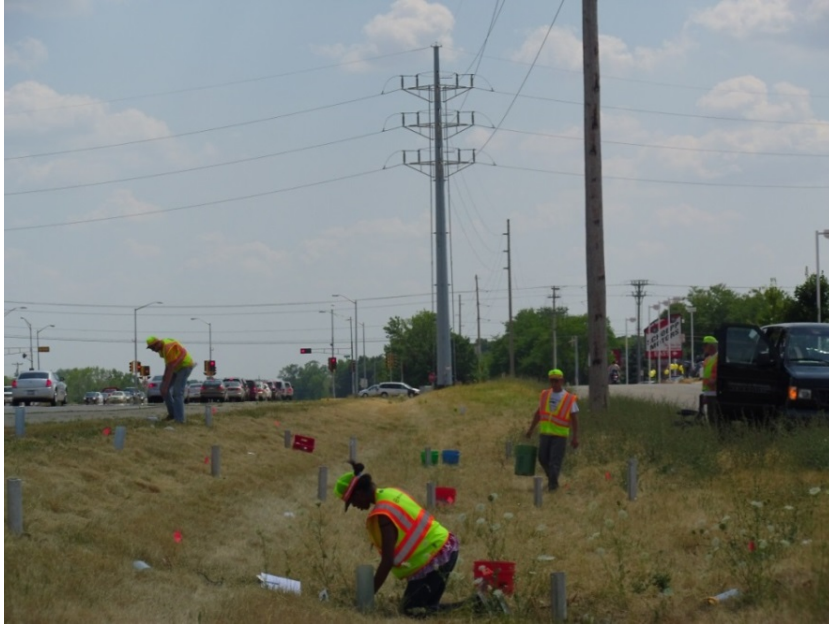
Figure 14. Taking infiltration measurements using the MPD Infiltrometer in the swale located near Hwy 51, Madison, WI.
