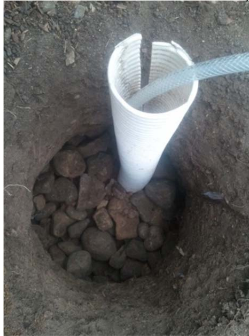
Figure A.1. Backfilling the hole during installation of the SPE20 sampler (white PVC used to protect the device during backfilling rocks at the Hamline-Midway site).
