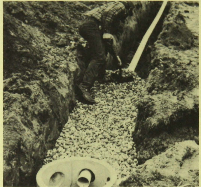
The drop box in the foreground directs effluent into the 4-inch pipe and the drainfield trench. Drop box distribution is especially effective for resorts, where sewage flow rate varies. Drop boxes allow the soil treatment unit to be easily expanded.
