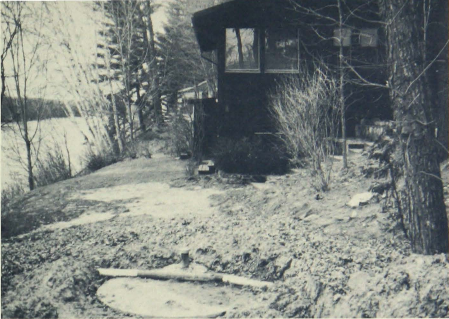
A holding tank is needed where the topography or the lot area does not allow installation of a soil treatment system.
