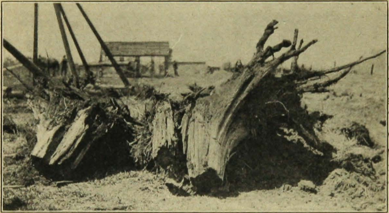
Fig. 3. White Pine Stump Pulled first then cracked with dynamite
