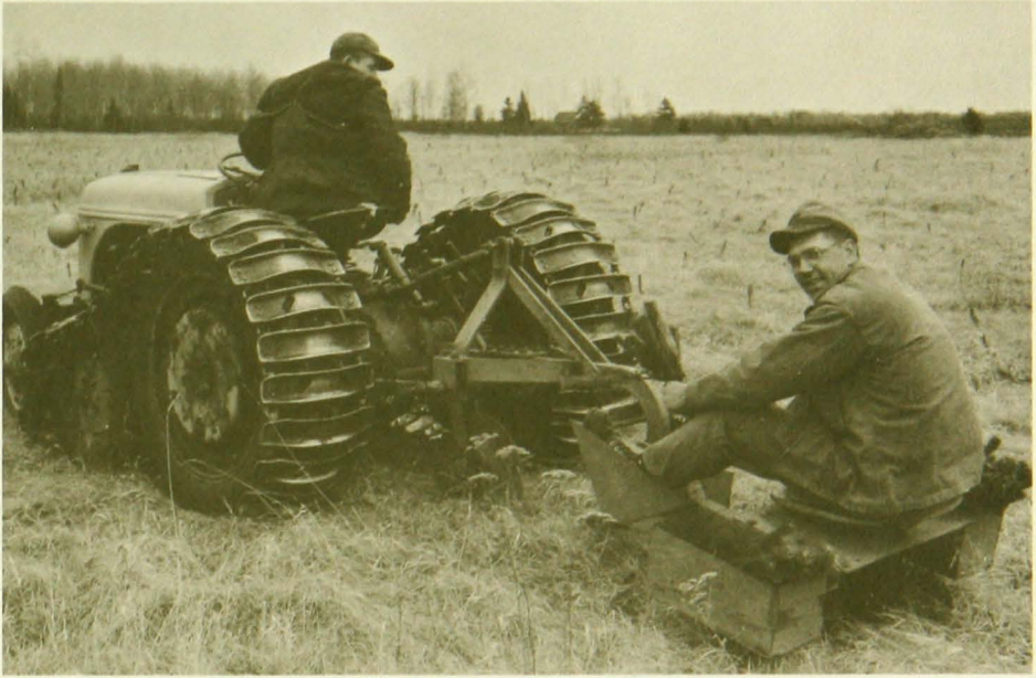
Figure 2. Three point hydraulic lift controls planting depth.
