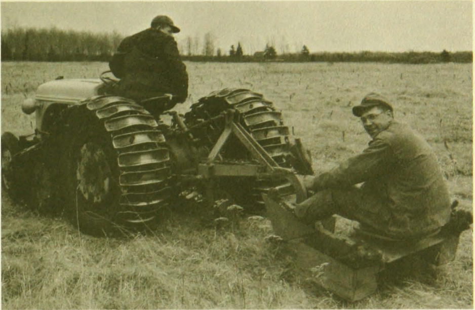
Figure 2. Three point hydraulic lift controls planting depth.
