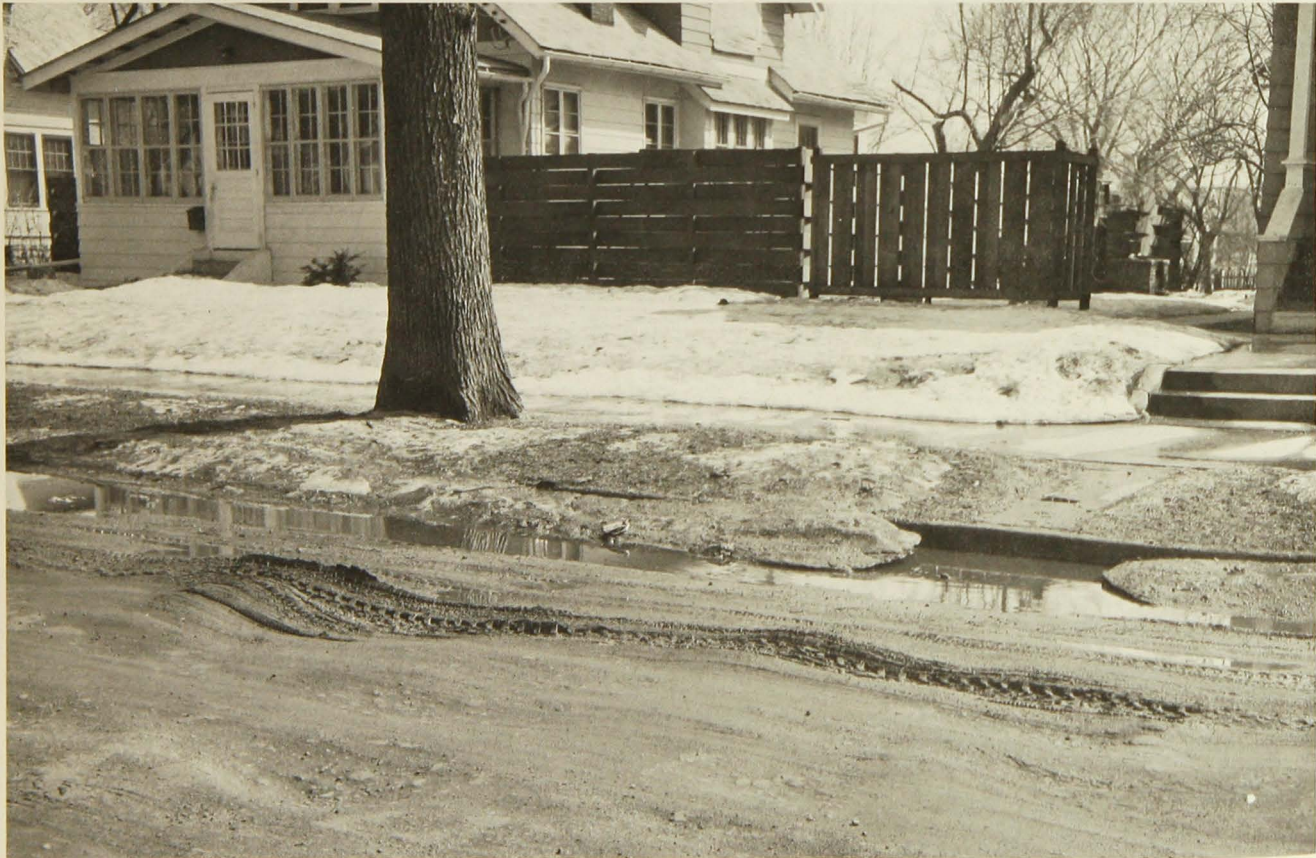
Figure 5. Organic and plastic soils provide insufficient bearing support for today's traffic loads.
