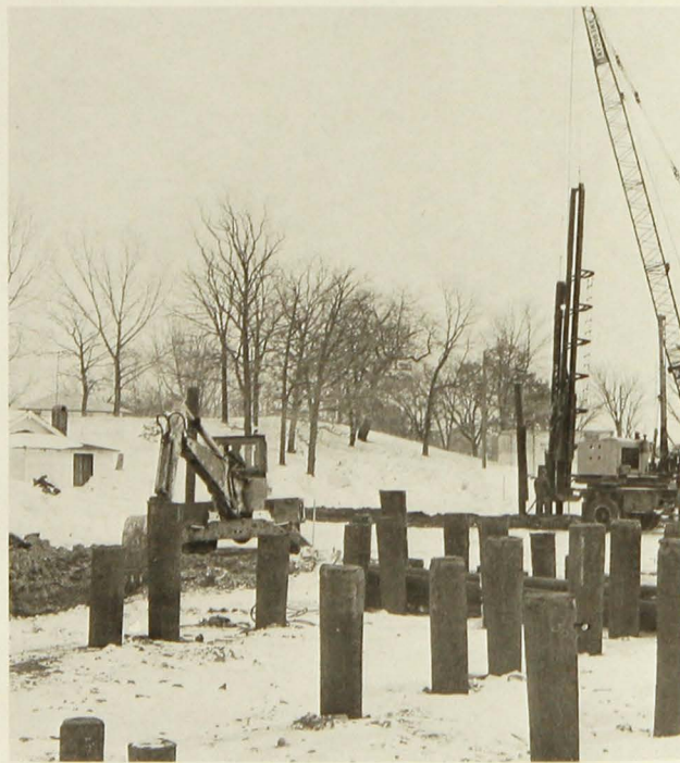
Figure 39. Piling driven to support an apartment building development on Group 6 soils near Lake Phalen, St. Paul. Development costs are high for building sites on these soils.
