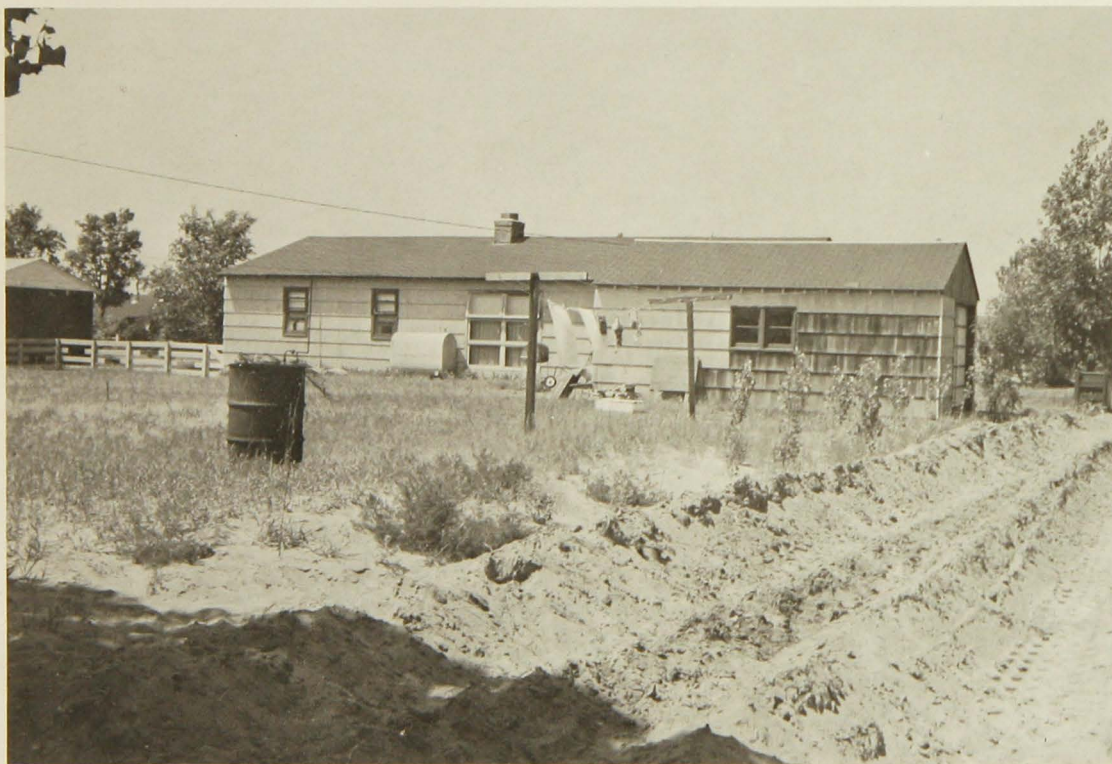
Figure 15. Sand blowing in a Group 1 soil area where vegetation had been removed caused this problem.
