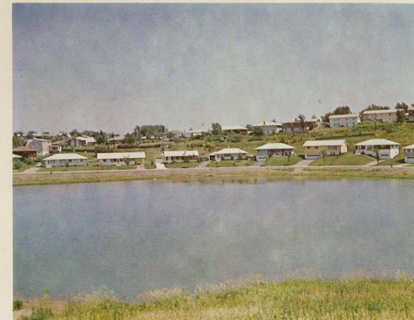
Figure 43. Shallow lagoon created in a poorly drained peat area handles surface water runoff and contributes to the residential setting.
