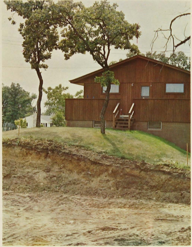
Figure 29. Undisturbed soil is preferred for building sites. Note difference in appearance between undisturbed natural soil profile at right and filled area at left. Both are in the same excavation.
