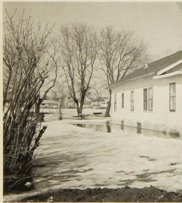
Figure 37. Poor surface drainage often results in frequent flooding of basements and can lead to rapid deterioration of buildings.
