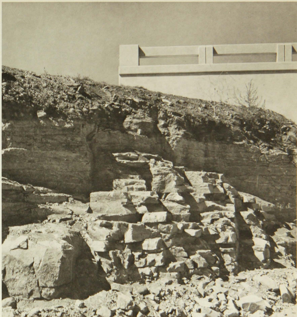
Figure 48. Excavation costs are increased when underlying rock of Group 8 soils is unweathered limestone.
