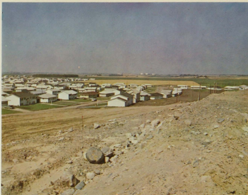
Figure 20. A new residential development on level Group 2 soil with gravelly, stony material typical of rolling soils of Groups 2 and 3 in the foreground. Underlying material of the level area consists of boulder-free sands and gravels.
