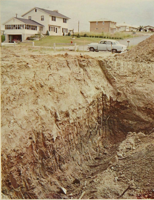
Figure 29. Undisturbed soil is preferred for building sites. Note difference in appearance between undisturbed natural soil profile at right and filled area at left. Both are in the same excavation.
