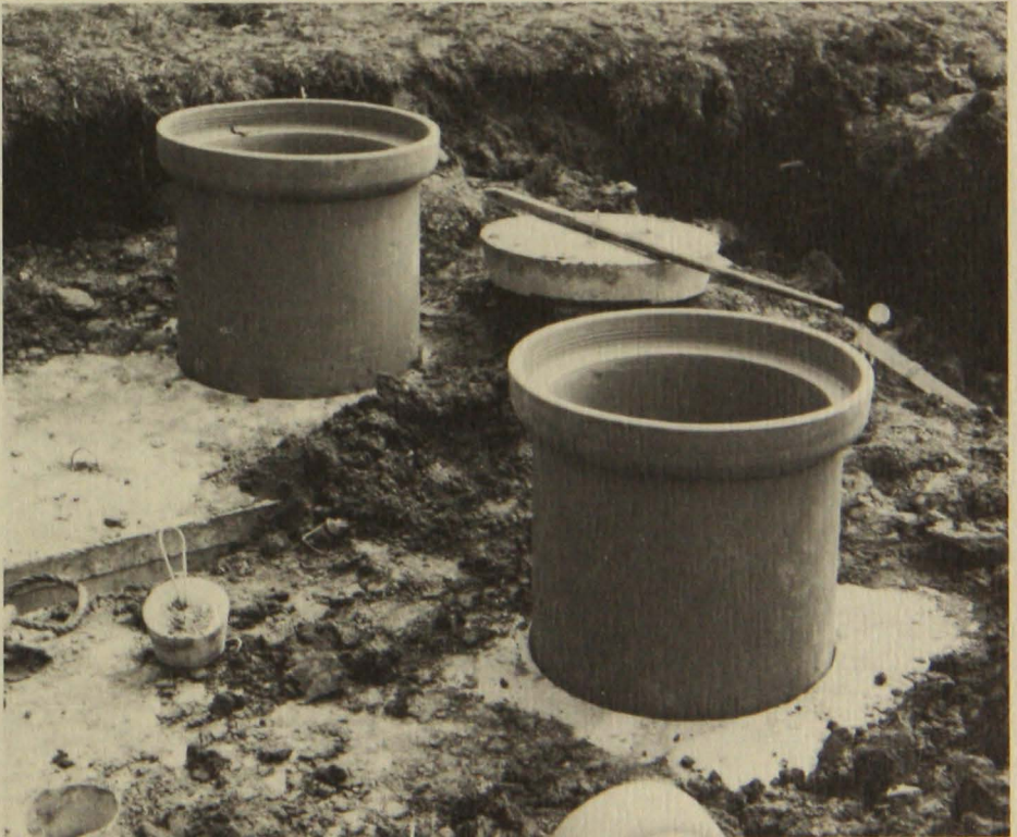
Manhole access is necessary for septic tank and pumping tank maintenance. The manhole cover should be secured to prevent unauthorized entry.
