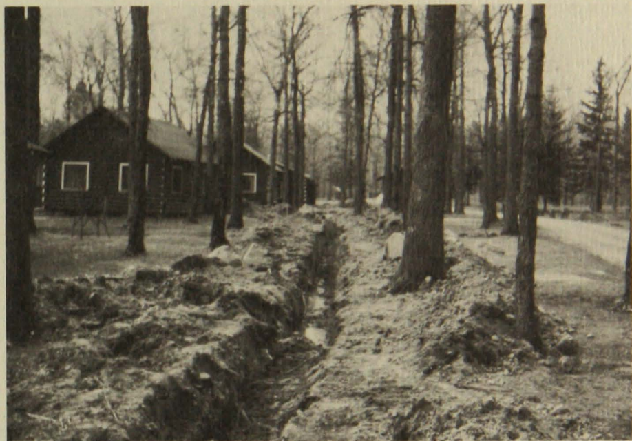
A collector sewer line for effluent serves these lakeshore cabins. Each cabin has its own septic tank.
