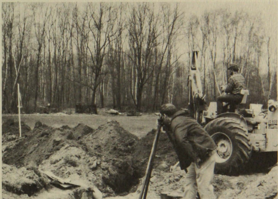
A tripod surveying instrument is essential for the sewage contractor. The trench bottom must be level through the length of the trench.
