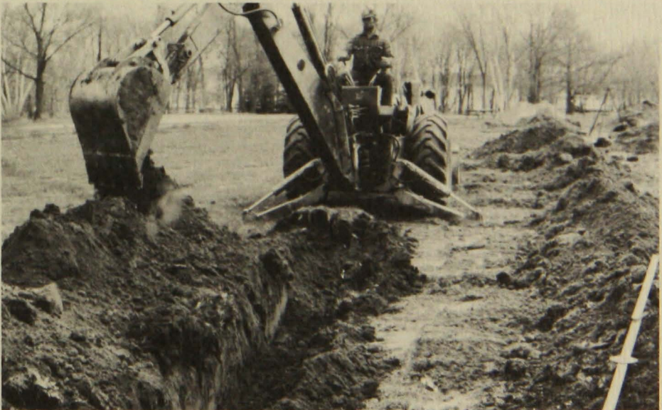
A back hoe is used to properly excavate drainfield trenches. Shallow trenches provide the most effective sewage treatment.
