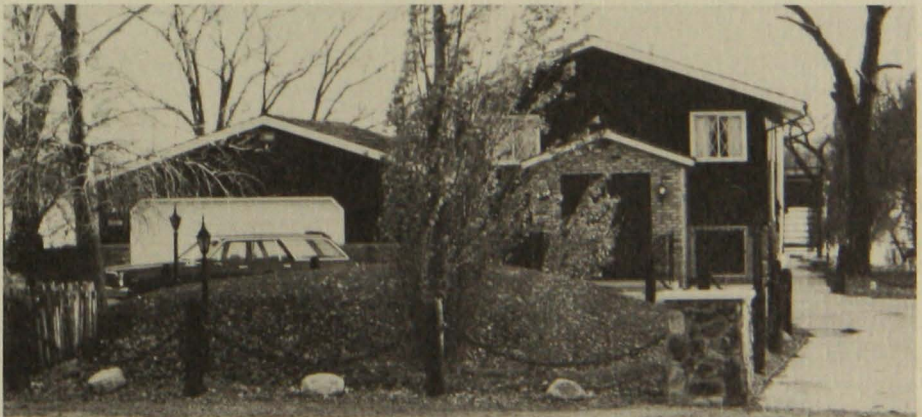
This completed sewage treatment mound might easily be mistaken for a berm commonly used in landscape architecture. The top of the berm is crowned to promote runoff of heavy rains. This berm adds interesting relief to an otherwise flat landscape and serves as a privacy barrier.
