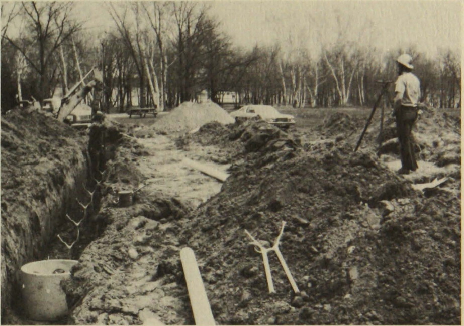
Pipe saddles installed in a drainfield trench hold the distribution pipe on a uniform grade. A tripod level is used to set grade for the trench distribution pipe which will connect to the drop box in the foreground.
