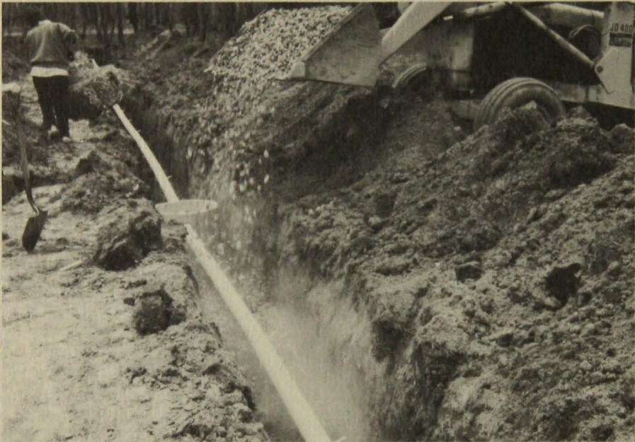
Clean rock placed carefully in the drainfield trench to avoid disturbing the distribution pipe supported at the proper grade. Note the drop box.
