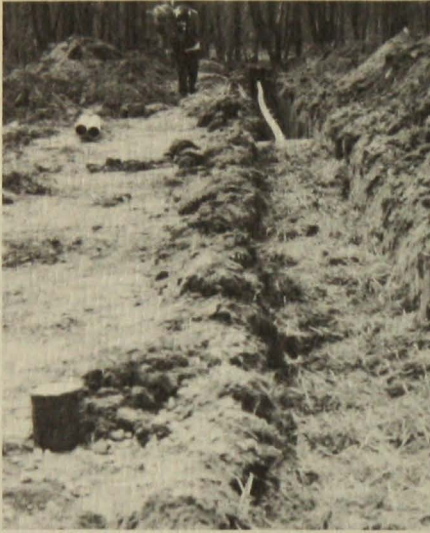
Hay or straw cover prevents soil backfill from filtering down into the trench rock.
