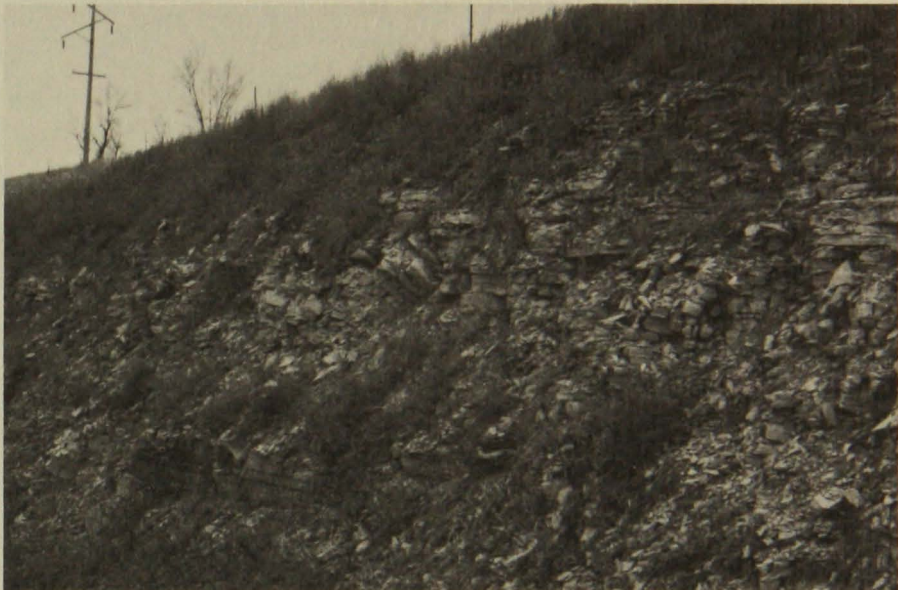
Fractured bedrock, like this limestone rock exposed in a highway grade, does not provide adequate treatment of sewage unless at least 3 feet of suitable soil exists between the trench rock and the limestone bedrock.
