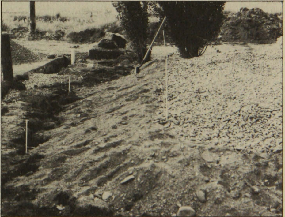
This sewage treatment mound under construction shows the roughened original soil covered with a 12-inch layer of clean sand. The layer of clean, \frac{3}{4} -inch rock is ready for placement of distribution pipes. Careful construction procedures are essential for successful mound performance.
