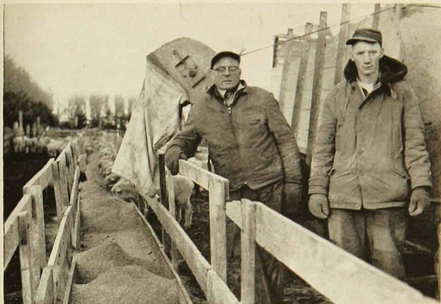
Fig. 5. "Mechanized" feeding can give an operator great flexibility in handling lambs on feedlot. This Minnesota farmer is using a self-unloading and mixing wagon, drawn by a tractor. The system is also practical in smaller-scale operations.
