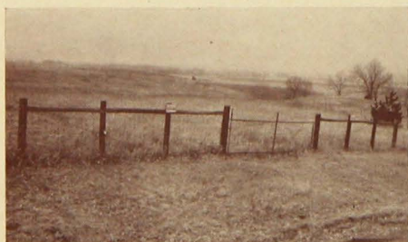
Conventional gate bracing (in service 12 years).
