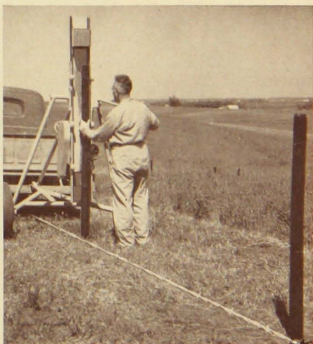
Power driving line posts.
