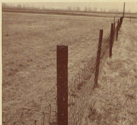
Posts on alternate sides of the wire (in service 8 years).
