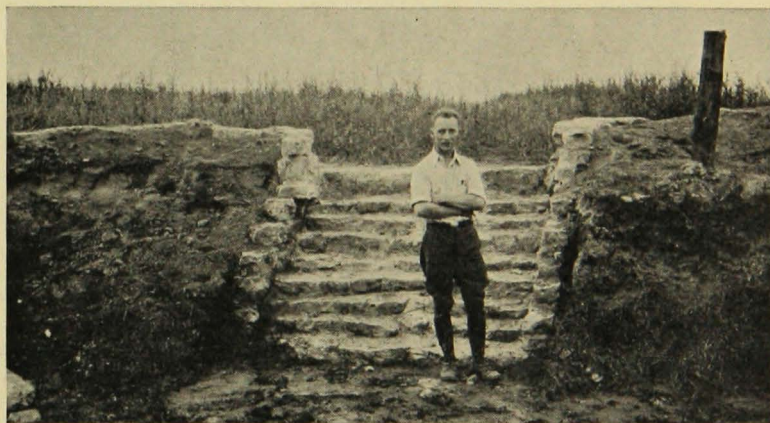
FIG. 15. AN EFFECTIVE TYPE OF TERRACE OUTLET BUILT OF RUBBLE MASONRY
