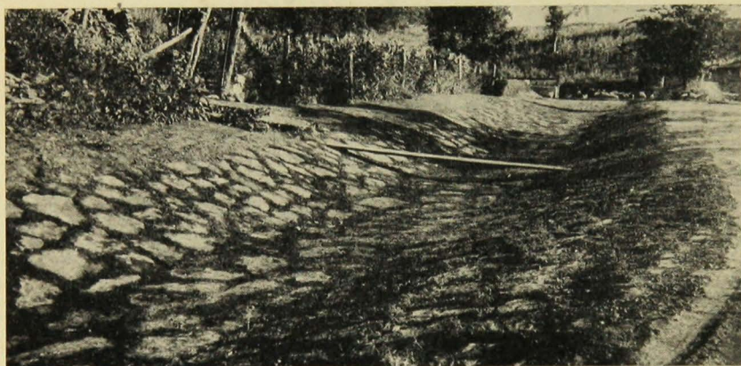
FIG. 13. TERRACE OUTLET PAVED WITH FLAGSTONES AND WITH THE SPACES BETWEEN THE STONES CALKED WITH SOD
