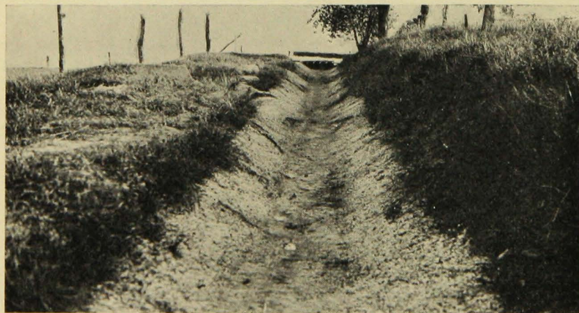
FIG. 14. TERRACE OUTLET PAVED WITH TARVIA
