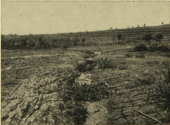
FIG. 27. A SERIES OF PROPERLY SPACED BRUSH DAMS THAT HAVE CAUSED A GULLY ORIGINALLY ABOUT SIX FEET DEEP TO FILL UP
