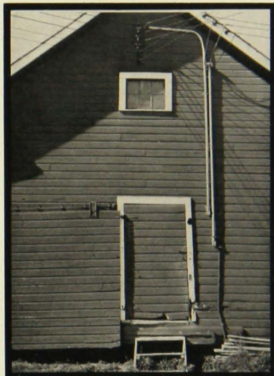
FIG. 13. MAIN SERVICE ENTRANCE SWITCH LOCATED IN THE GRANARY
