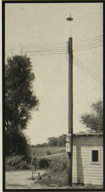
FIG. 10. SERVICE POLE WITH YARD LIGHT
