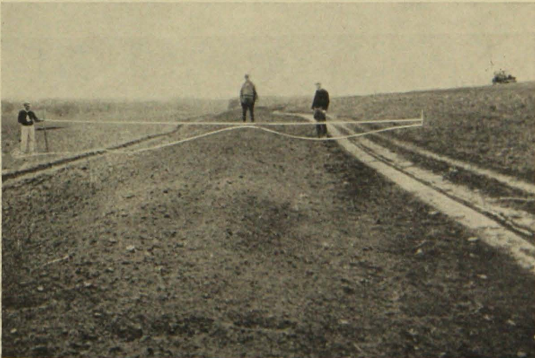
Fig. 10. Terrace Built by the Iowa Terracer (Courtesy Agricultural Engineering Department, Iowa State College)
