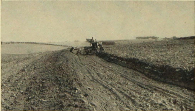
Fig. 12. Terrace Built by the Missouri Terracer (Courtesy of the Missouri Station and "Agricultural Engineering")
