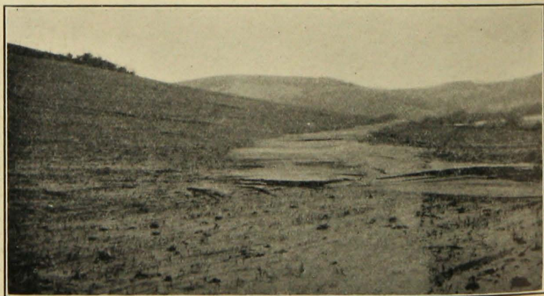
Fig. 8. What became of part of the silt washed from the slopes shown in Fig. 7. A large diversion ditch was completely filled and rendered ineffective by the single storm because there were no other protection works on the slopes above it.
