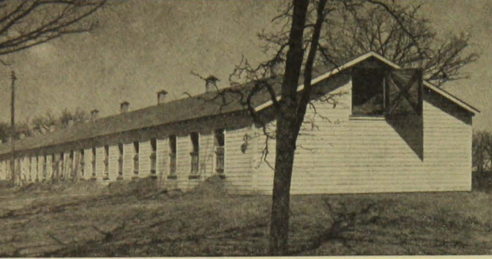
FIG. 4. A long straw loft house with roof vents
