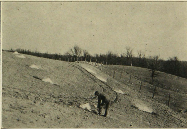
Fig. 10. Spreading Limestone with a Shovel from Half-Bushel Piles 24 Feet Apart
