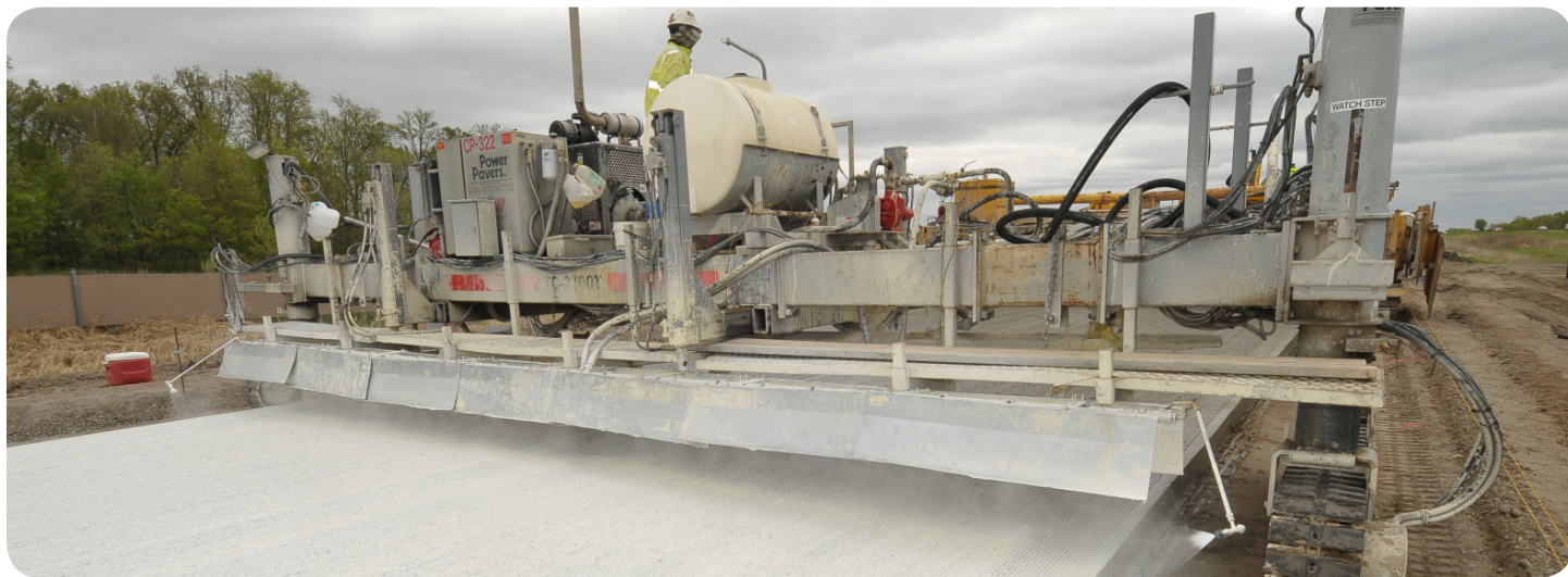
Construction of a concrete test cell at the MnROAD pavement research facility
