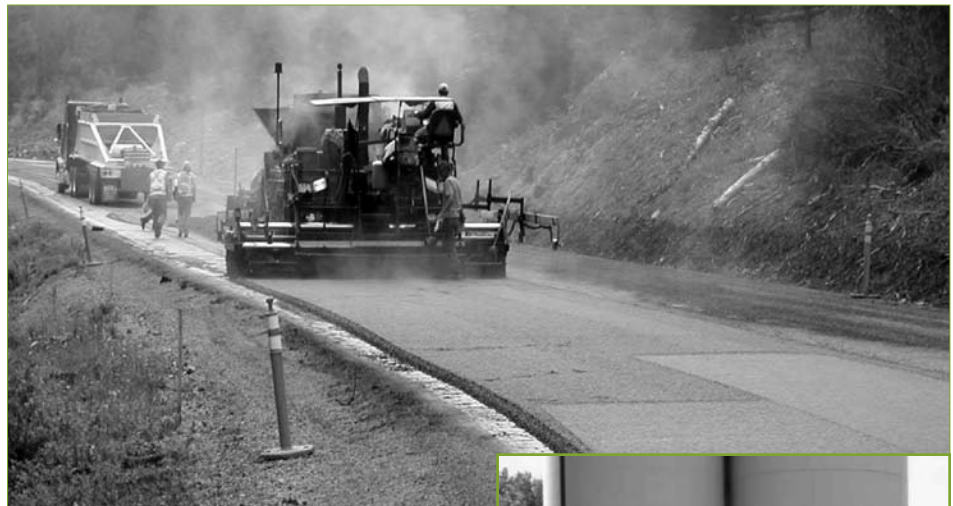
Figure 1: Conventional asphalt mix placed at 320° F.
