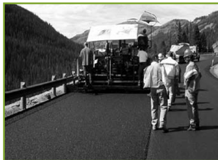
Figure 2: Asphalt with Advera additive placed at 245° F.
