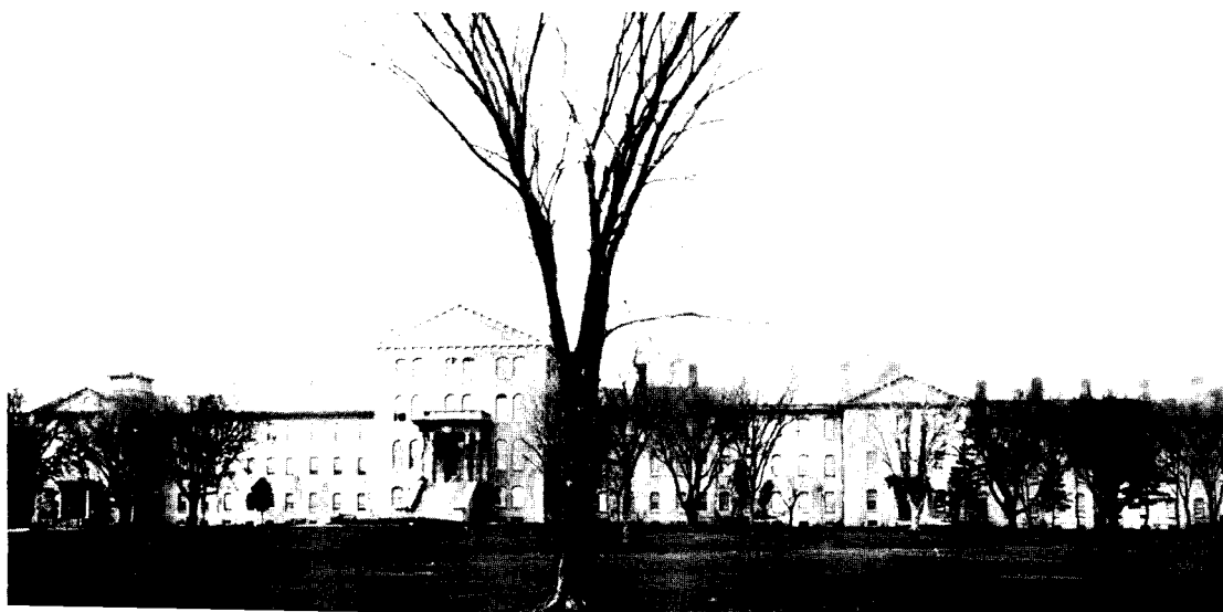
Old St. Peter State Hospital, Main building
