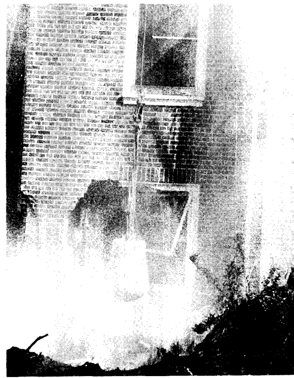
Demolition of Powell Hall and adjoining structure. (Story, Page 7)
