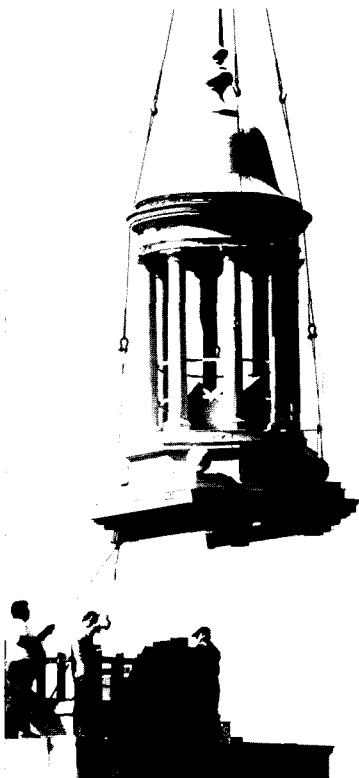
WORKMEN UNHINGE the cupola atop Powell Hall, the former nurses dorm on the Minneapolis campus, before the building was demolished to make way for a new University Hospitals facility.
