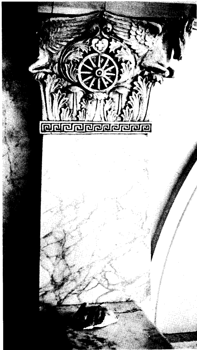
A souvenir hunter broke off a corner of a pillar and then decided to leave it behind.
