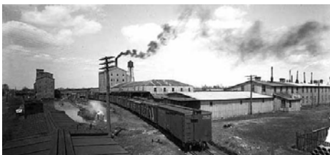
Figure 24 – Train yard from west
