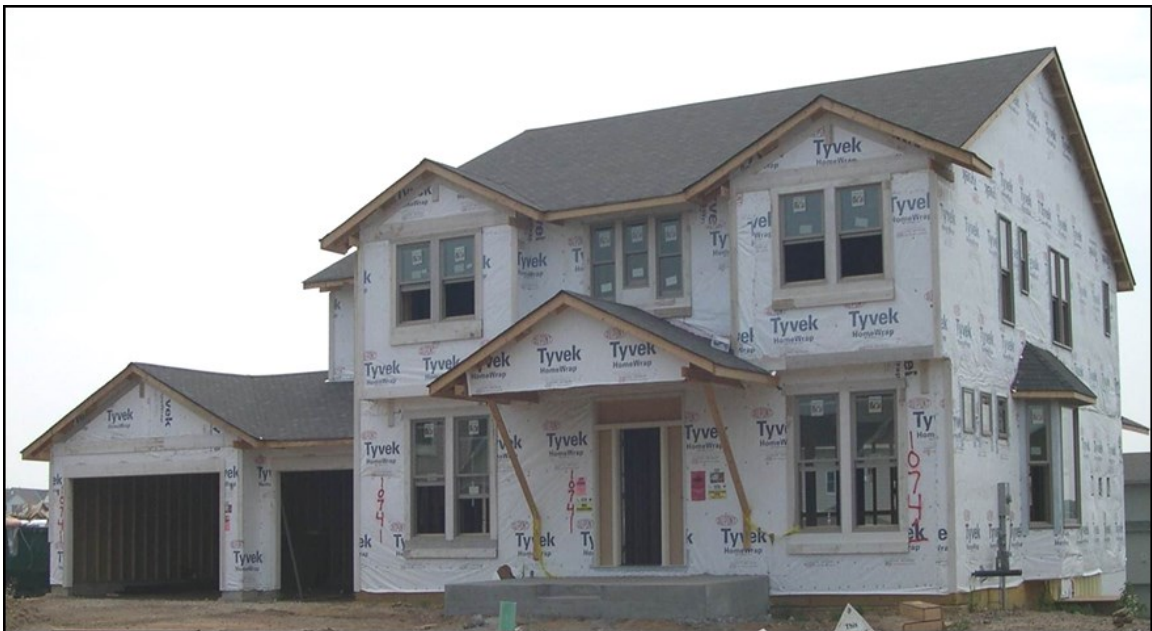
Figure 1. Cantilevered second story floors and cantilevered bay window
