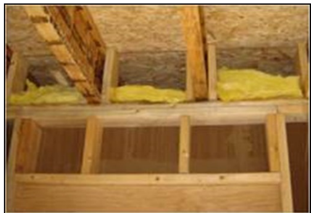
Figure 8. Cavities partially filled with batts
