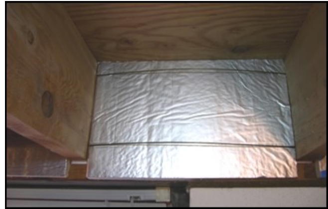
Figure 25. Temporary foam board blocking
