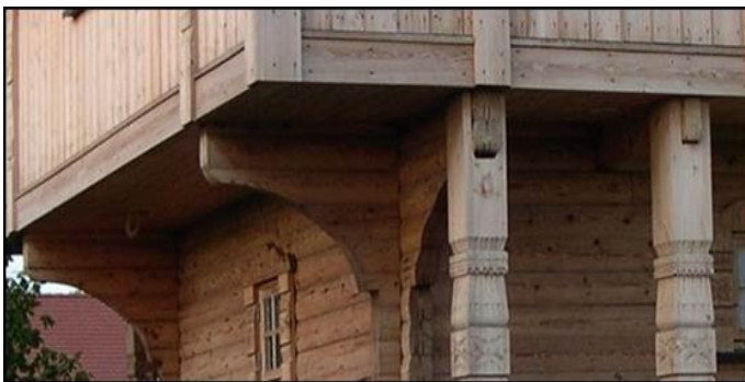
Figure 6. Uninsulated timber floor in Green Lake, WI
