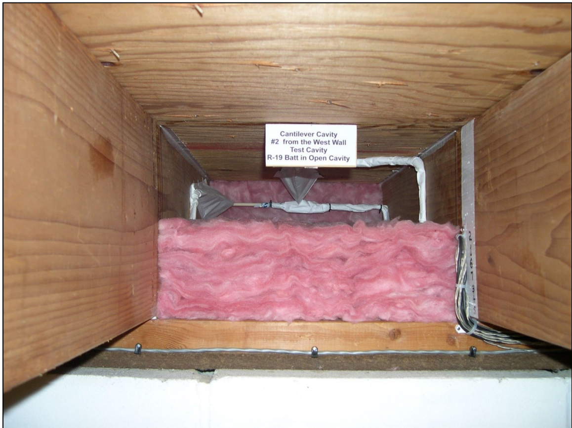
Figure 48. Completed R-19 test cavity
