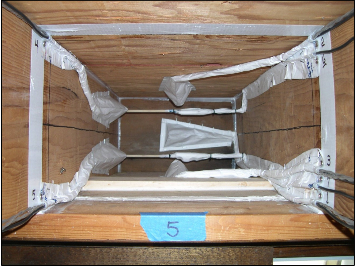
Figure 43. Soffit cover installed. Sensor group enclosures and cable covers attached
