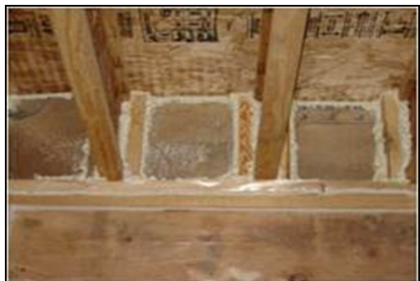
Figure 11. Cavities blocked and air-sealed
