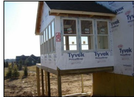
Figure 3. Attached sunroom on piers
