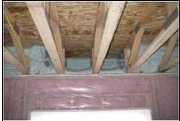
Figure 9. Spray applied polyurethane foam
