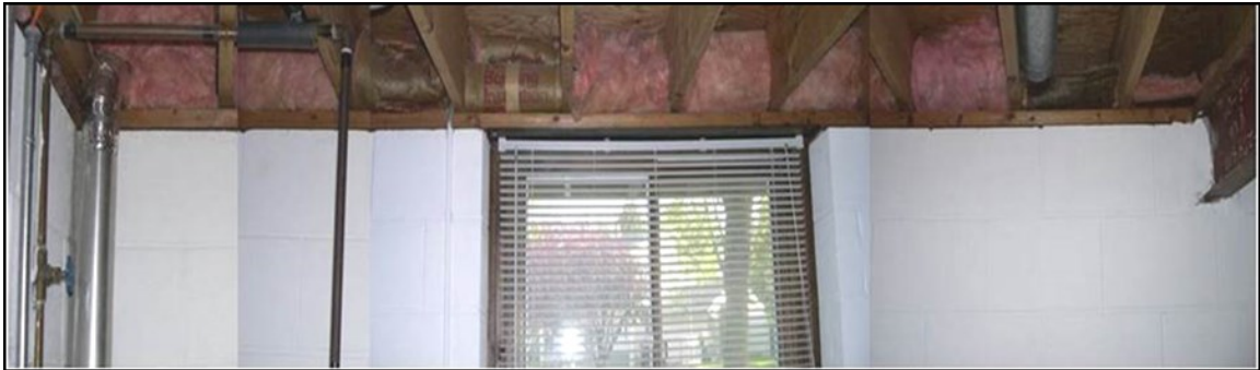
Figure 17. Interior of the cantilever in 'as found' condition (west side)
