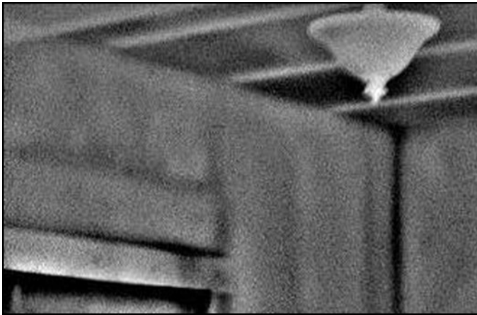
Figure 12. Thermograph of cold ceiling surfaces below the cantilevered floor
