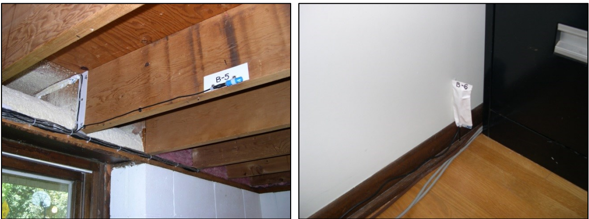
Figure 51. Boundary sensor-basement location Figure 52. Boundary sensor-main floor-west
