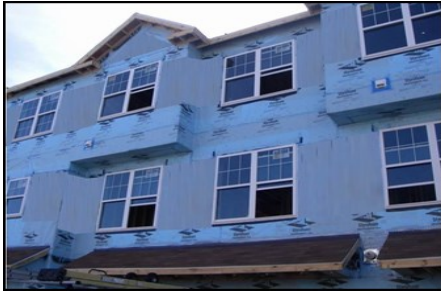
Figure 2. Multi-family housing with cantilevered third story floors
