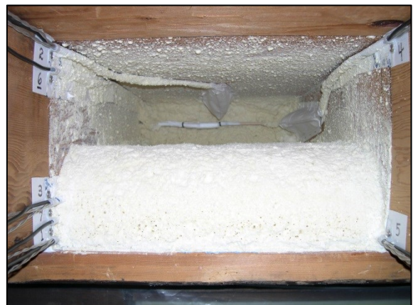
Figure 47. Masking removed from enclosures
