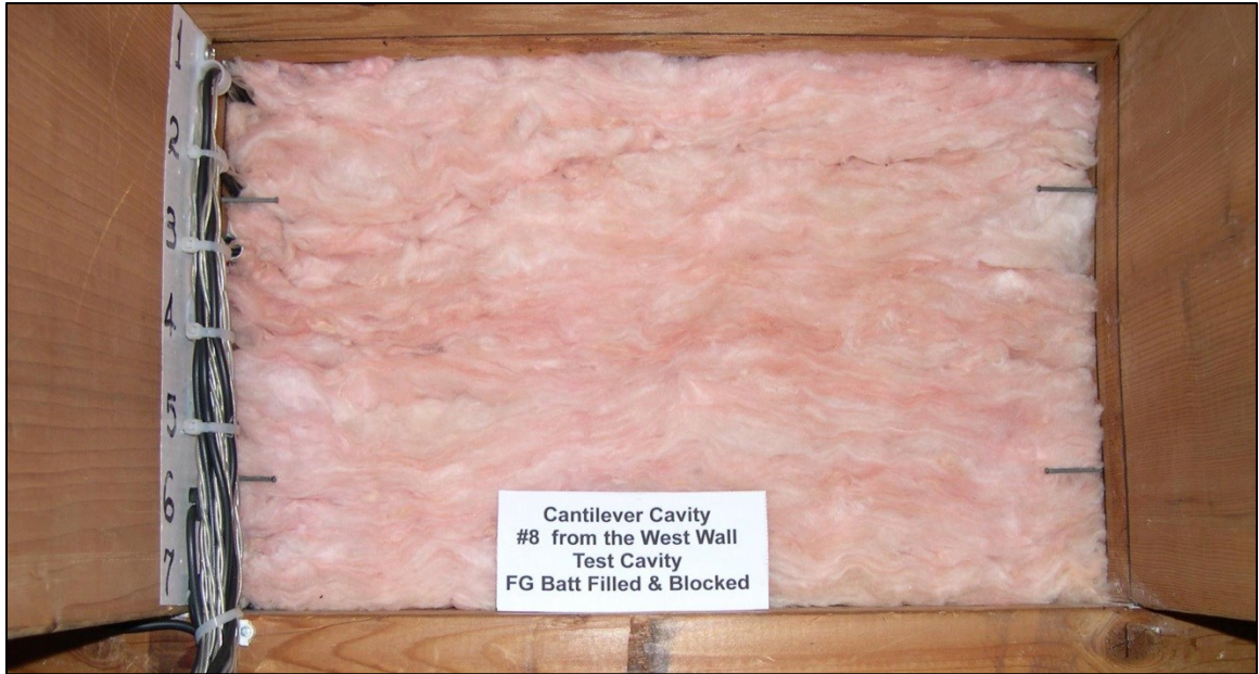
Figure 49. R-30 insulation fill completed
