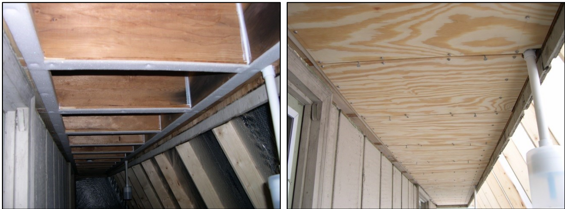
Figure 33. Shimmed, sealed, and gasketed
