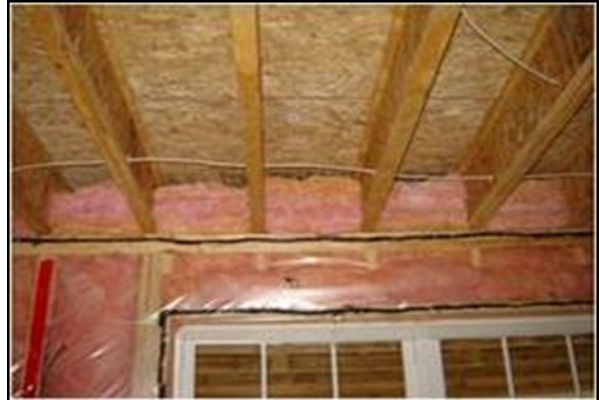
Figure 10. Cavities filled completely with batts
