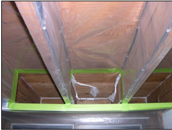
Figure 44. Masking for foam installation
