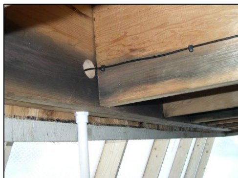
Figure 32. Housing and cable installed
