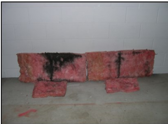
Figure 23. Evidence of infiltration through the cantilever assembly
