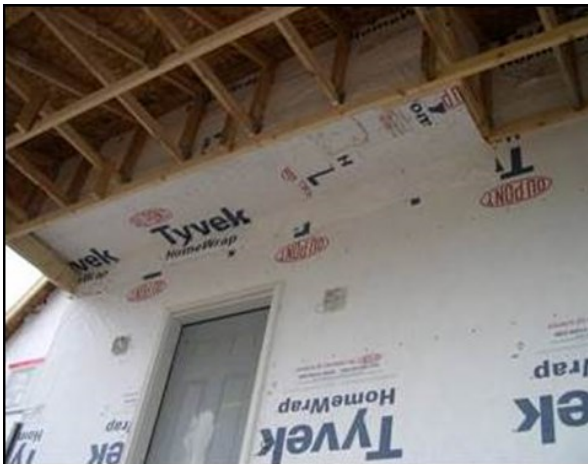
Figure 7. Exterior view of cantilevered floor during construction
