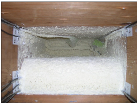
Figure 46. Enclosures masked outside foam fill
