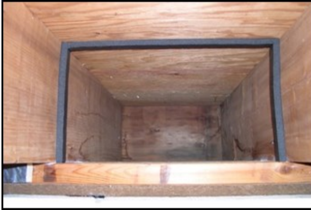
Figure 24. Temporary foam tape seal
