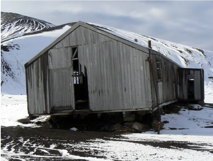
Figure 9. The Hunting Lodge has significantly less deterioration than other structures at the site partly due to a high foundation keeping the wood well above the soil. However the left corner shows erosion of the foundation that is in danger of collapse.
