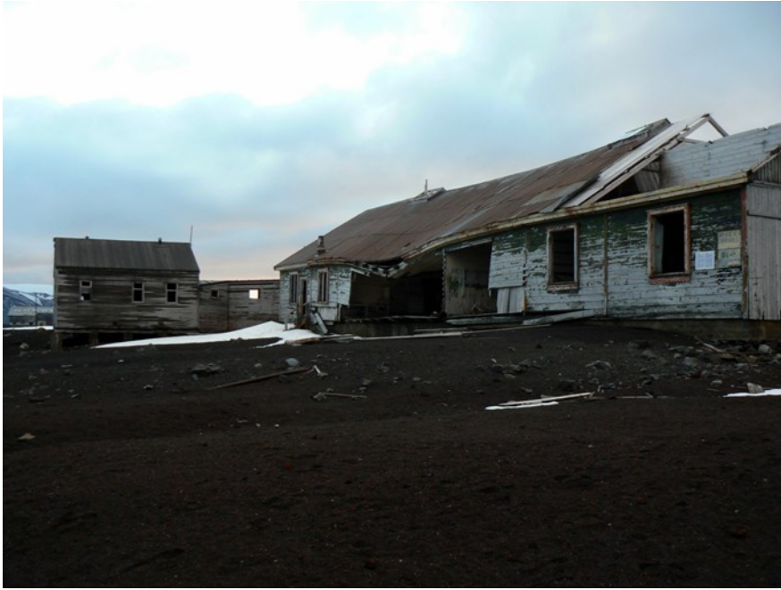
Figure 2. Structures at the whaling station at Whalers Bay, Deception Island are deteriorating. In addition to historic structures, there are a number of other wooden artifacts and equipment from the whaling period as well as activities by the British Antarctic Survey located on the island that are also decaying rapidly.
