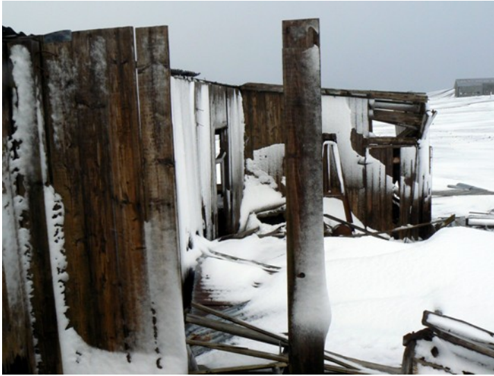
Figure 7. The north side of the dispensary at the end of a precipitation event showing accumulation of snow sticking to the wall boards. When this snow melts it is sufficient moisture to support fungal growth and decay.
