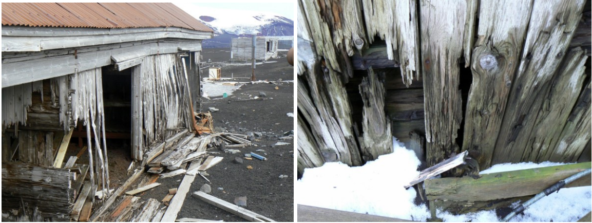
Figure 3. Left: The north side of the Biscoe House showing advanced decay of the wall boards. Right: Decay is occurring in many areas well above the soil line, as shown in these wall boards of the dispensary structure.
