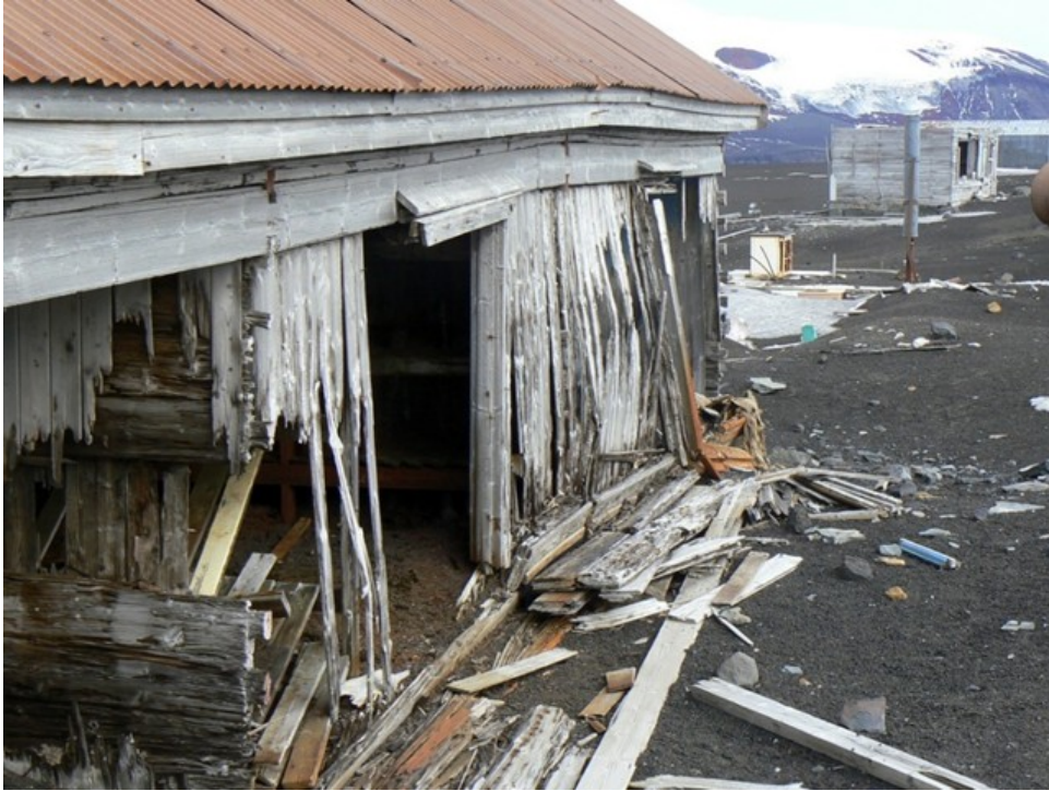
Figure 4. The side of the Biscoe House, a building at Whalers Bay on Deception Island, showing extensive decay of wall boards and other timbers.
