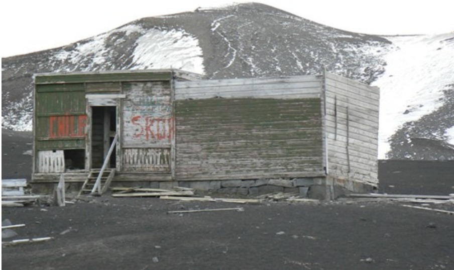
Figure 4. The Magistrate's residence has a solid foundation that has aided in avoiding deterioration by keeping the structure well above the soil. However, the roof has blown off exposing the interior to moisture.
