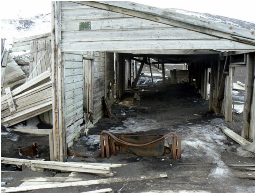
Figure 8. The dispensary/store has been inundated with mud from a lahar. The mud holds moisture and microbes which creates a conducive environment for decay to take place.
