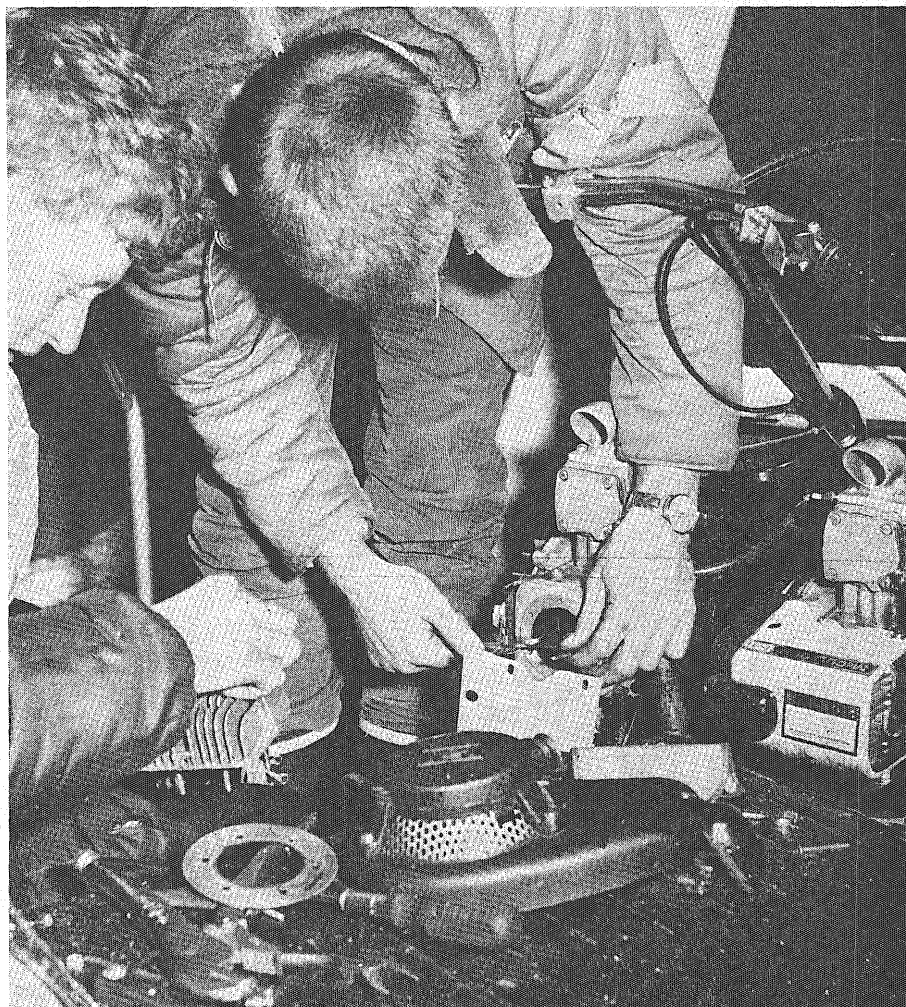
Below: After winning a race the United States Snowmobile Association official mikes the bore, checking the displacement of the engine. Above: Most snowmobiles come equipped with Rockwell JLO engines.
