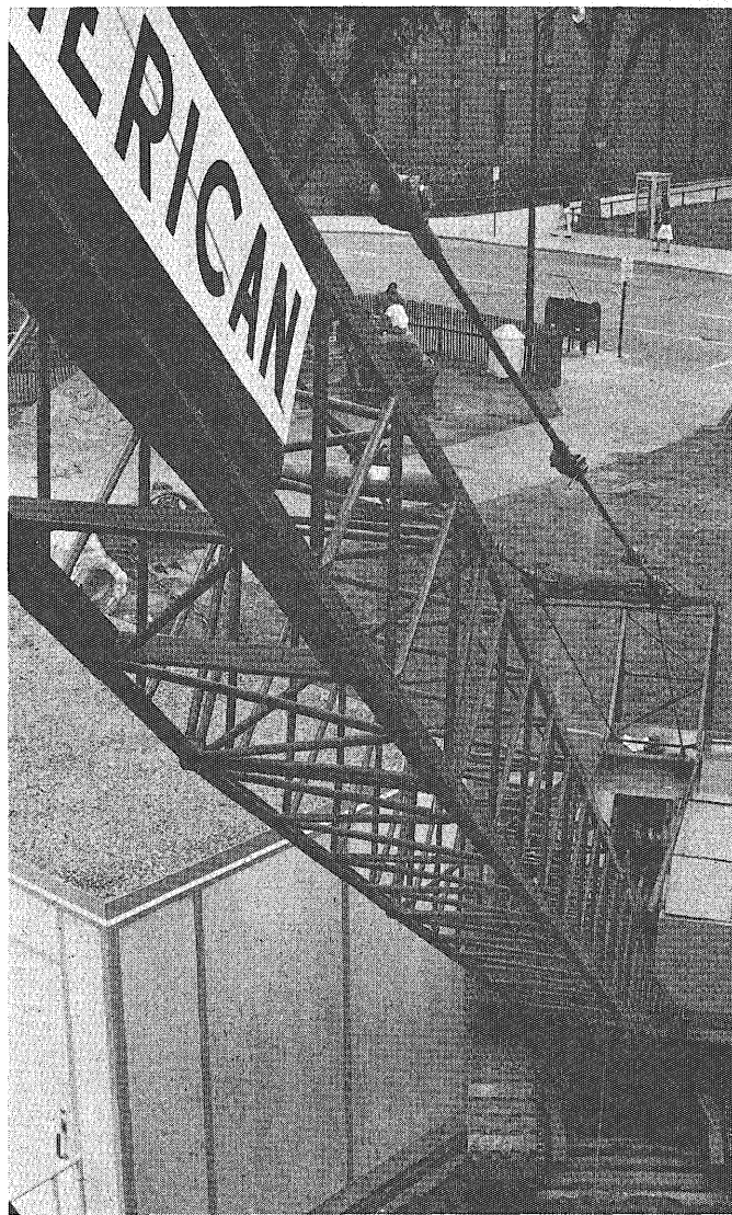
Crane is used here to wreck shaft of old freight elevator on north side of building. End of building at bottom was removed by cutting torch to make way for new addition.
