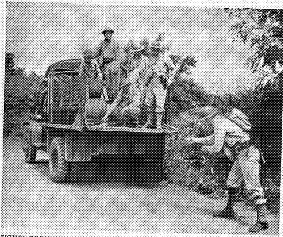
SIGNAL CORPS WIRE CREW laying wire for telephone communication. Wire can be recovered rapidly by the crew using a motor-driven reel mounted in the truck.
