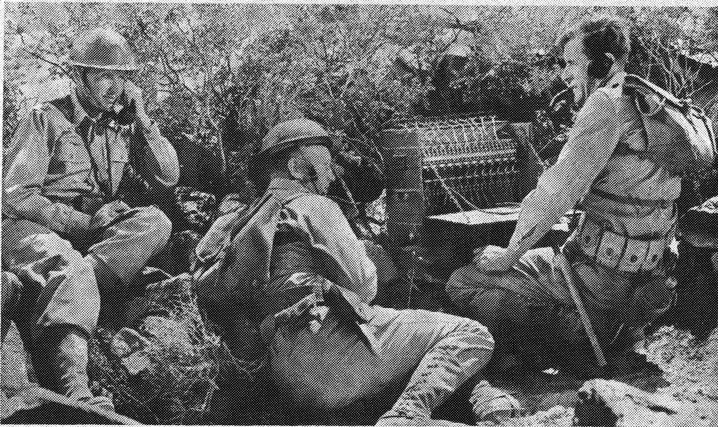
HIGHLY PORTABLE SWITCHBOARDS such as the one shown facilitate flexible communication between front line units during battle.
