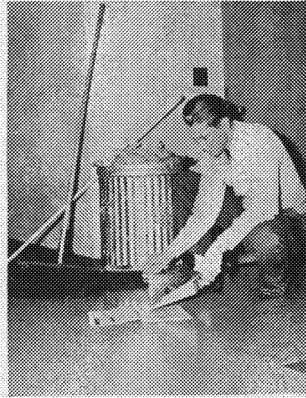
COLUMN NEEDS DIRT
