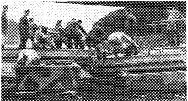
"... ponton bridges of various sorts are used ..."
