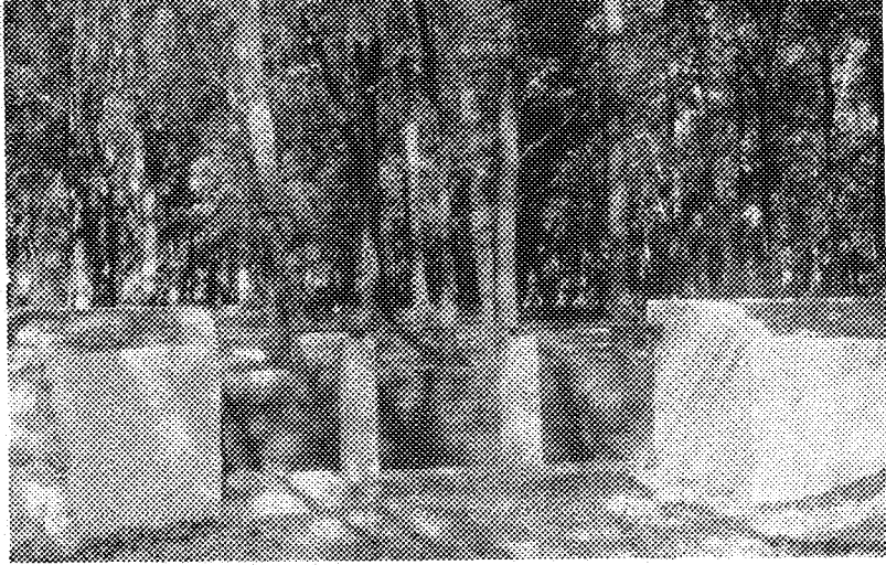
A dam erected to save a stand of trees by raising the ground-water level.
