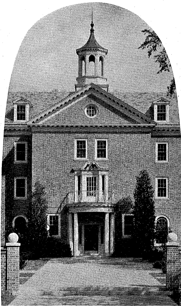
MAIN ENTRANCE — HALL
