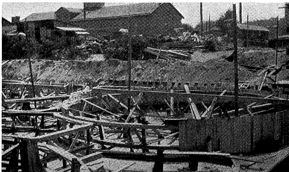
This form under construction shows the steel truss across the center and the method of placing the circular beams and of fastening the sides of these beams.
