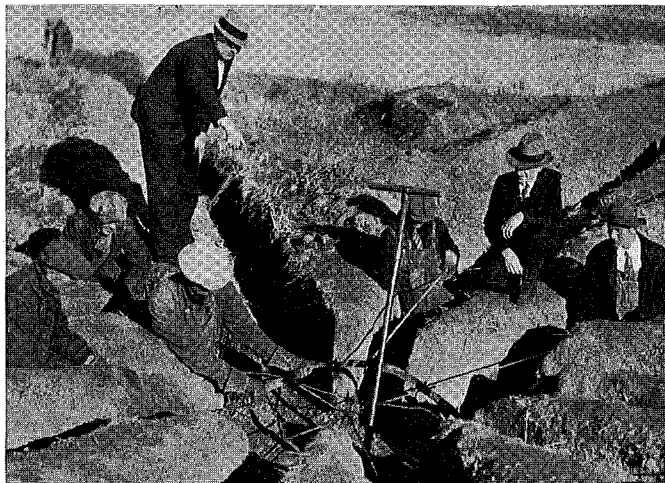
WORKMEN INSTALLING THE NETWORK FOR GROUNDING THE STATION
