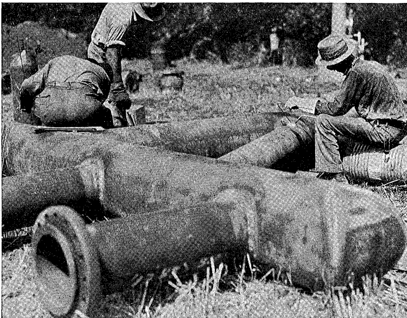
Welding a header. Special shapes such as this may be welded above ground and then moved into place. This practice is economical
