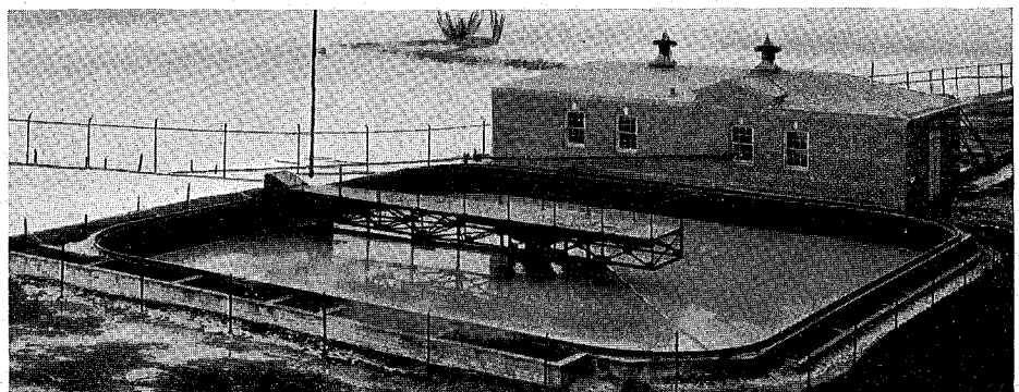
The building housing the plant is placed between the primary and secondary filters
