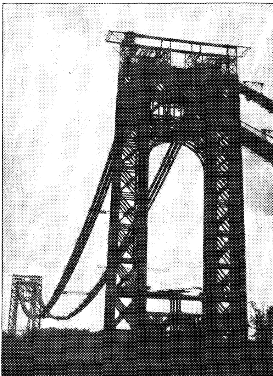
The Hudson River Bridge as it appears under construction.
