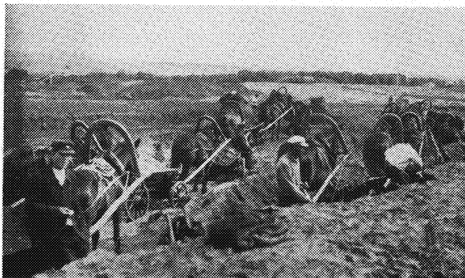
GRADING FOR A RAILWAY TERMINAL SHOWING ANTIQUATED EQUIPMENT.
