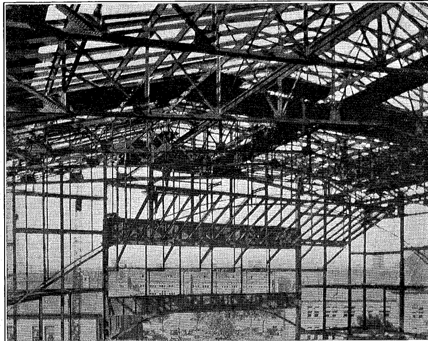
ROOF TRUSS CONSTRUCTION
