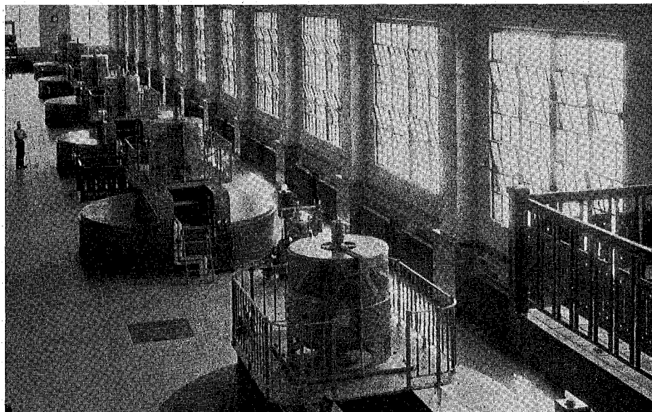
INTERIOR OF THE POWER HOUSE
