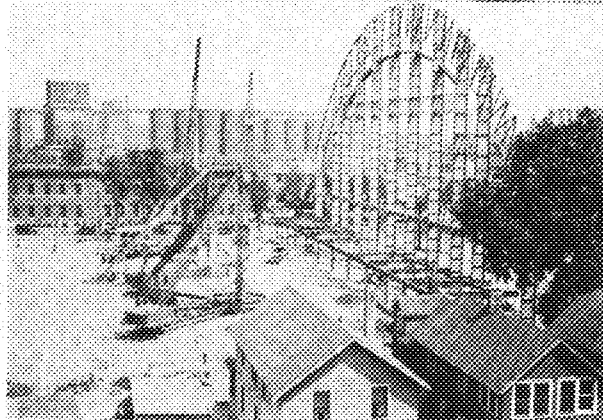
In the center picture is shown the process by which the arches are raised into place after being partly assembled on the ground. This type of erection is somewhat novel.
