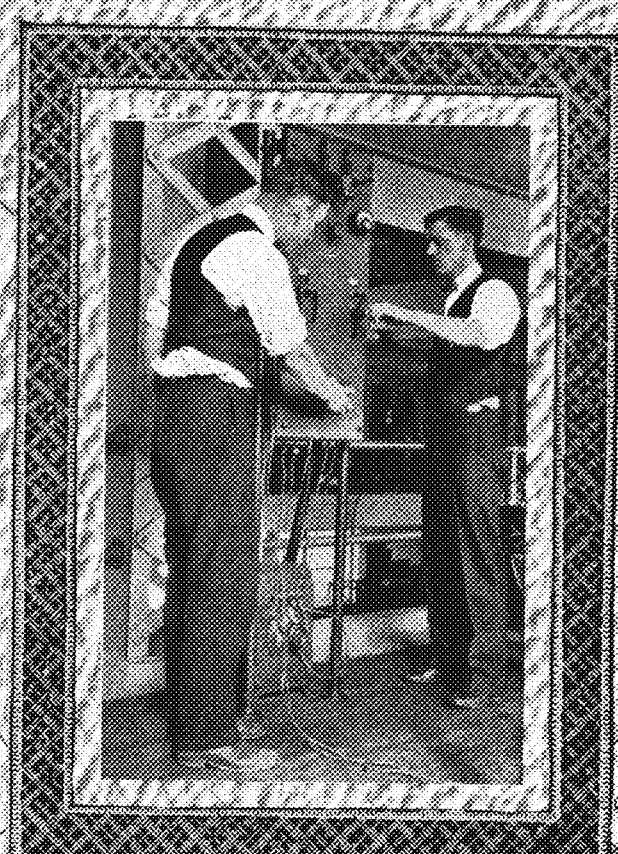
Electricals Test Mercury Arc
